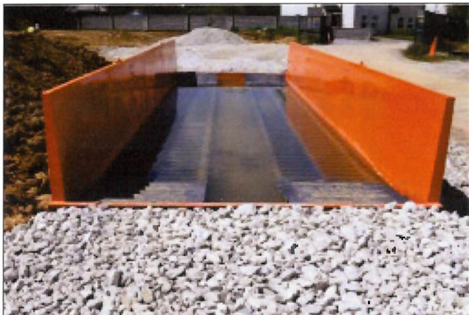
Figure 3: Stone access ramps in place
