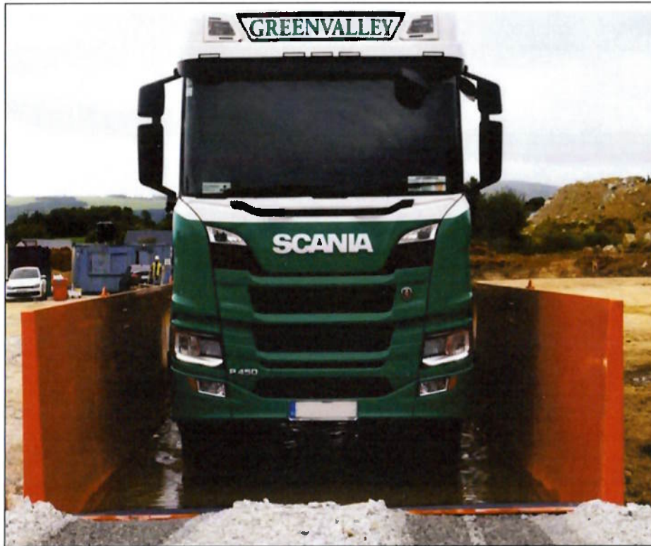
Figure 2: Eco Bath in use. Rumble tracks submerged in water
