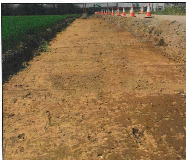
Plate 5 Topsoil Stripped Area (Sheet 1 Area)
