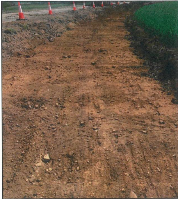
Plate 7 Topsoil Stripped Area (Sheet 2 Area; existing junction)
