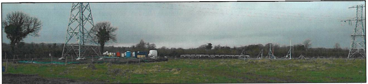
Plate 4 View from Substation Site Area looking west with temporary hardstand carpark in background and new masts to left and right
