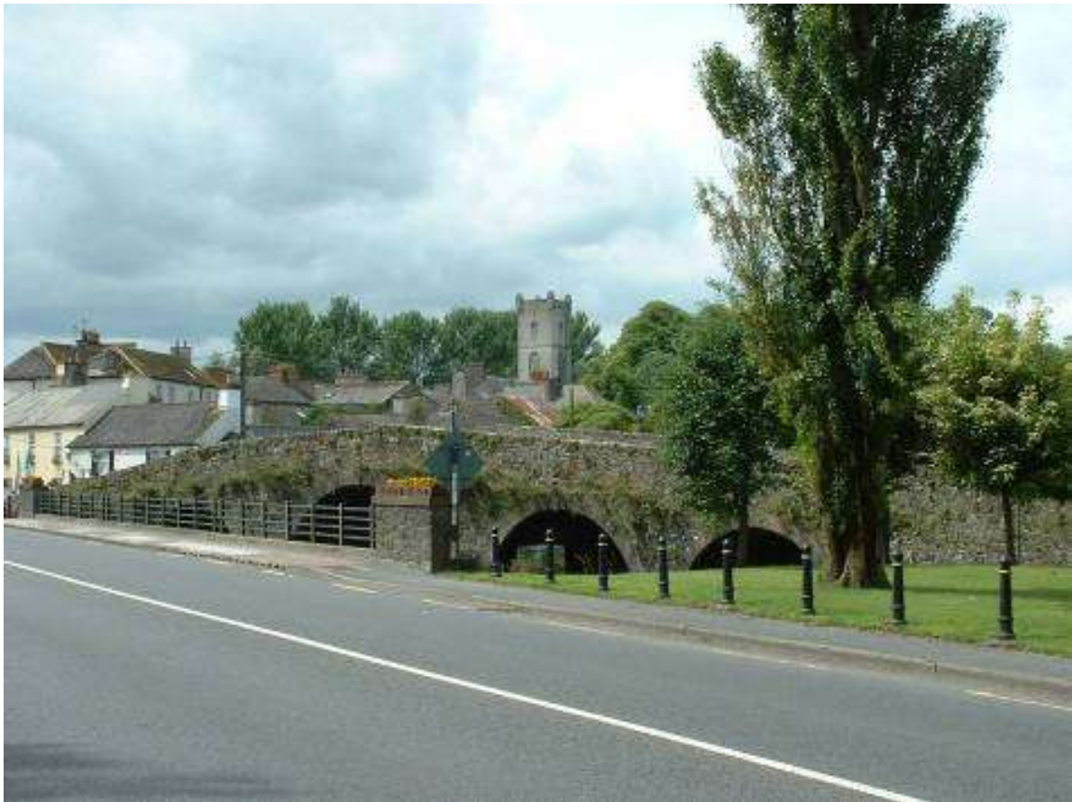
Figure 47. The Old Stone Bridge dating from 1788 over the Erkina River in Durrow
