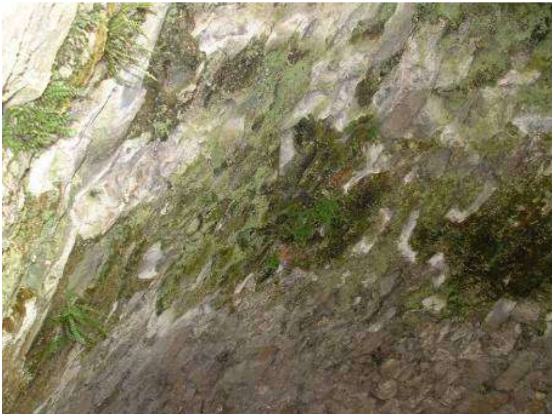
Figure 48. Underside of the Old Stone Bridge (BL1B) supporting ferns, lichens, liverworts and possibly bats.
