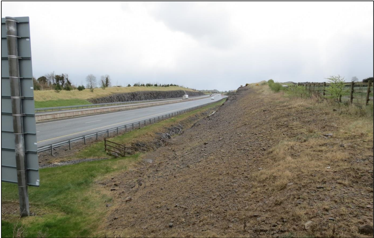
M7 Road Cut viewed looking east, beside M7 Motorway road sign.
