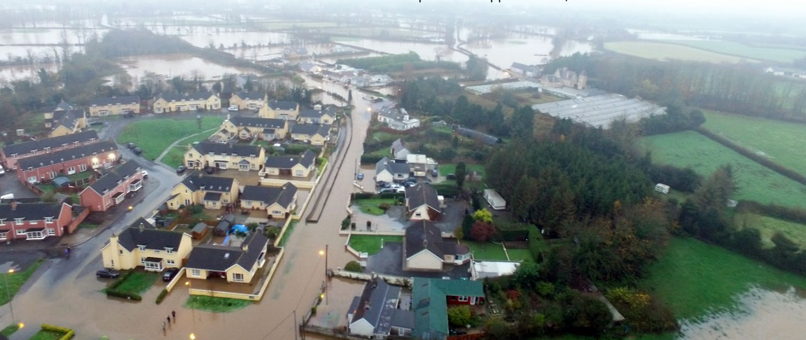
Flooding In Mountmellick in November 2017
