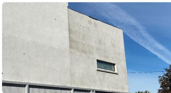
Swift bricks installed in the new library thanks to the work of BirdWatch Ireland (Laois branch) and Laois County Council
