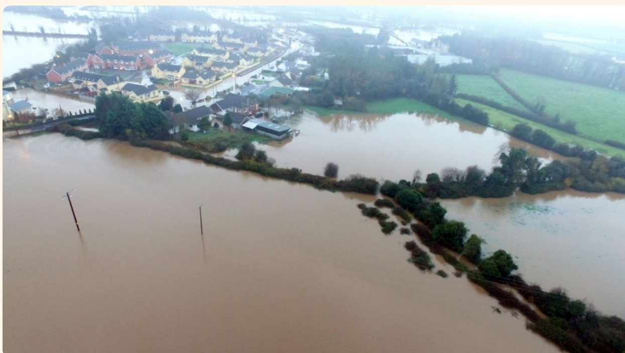
Flooding In Mountmellick in November 2017
