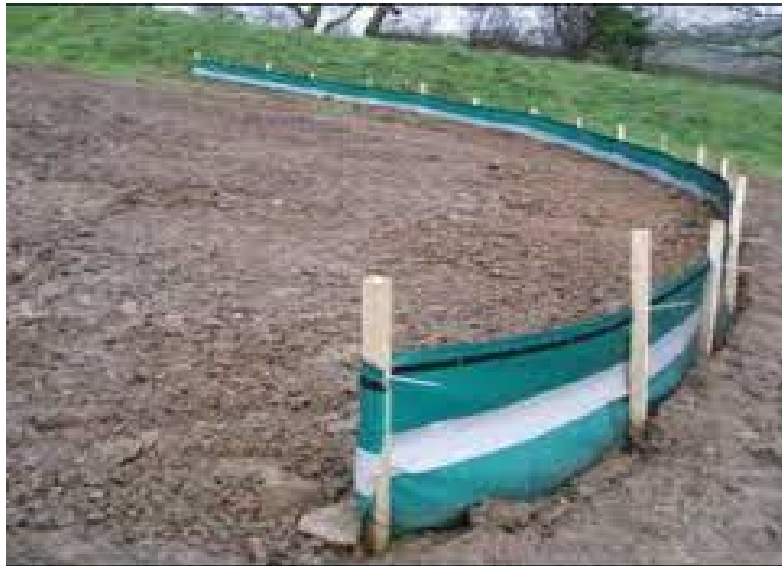
Figure 8: Silt Fencing
