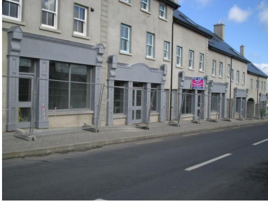
Good quality shopfronts on new shop units
