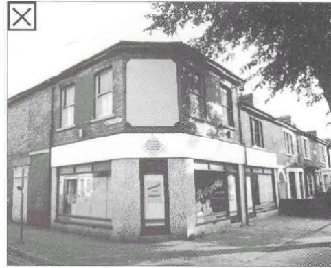
Poor quality use of materials can detract from the area as a whole
