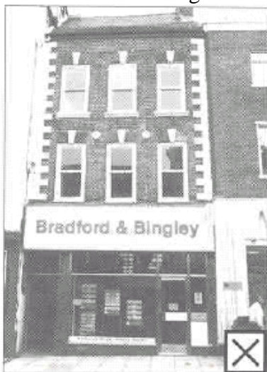
Inappropriate, oversized Fascia
