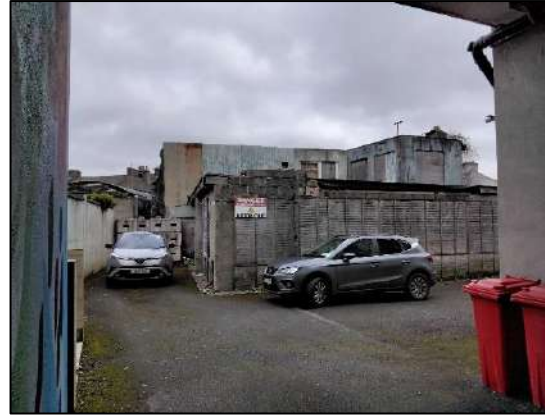
Plate 3-2 Exterior rear view of derelict structure.
