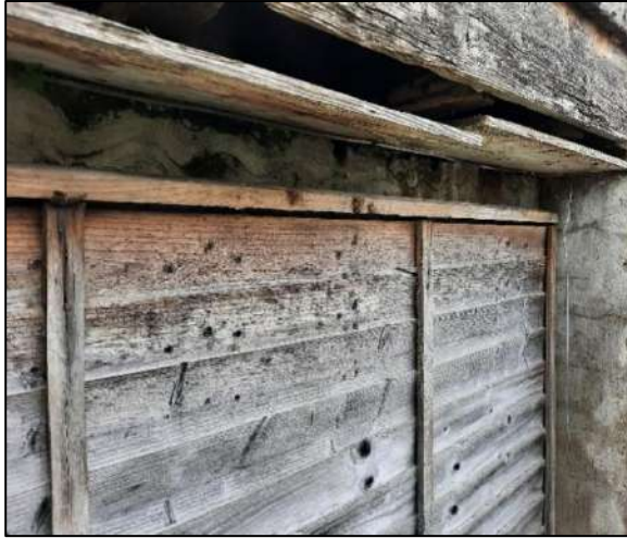
Plate 3-17 Facia of the rear structure showing bright light access internally.
