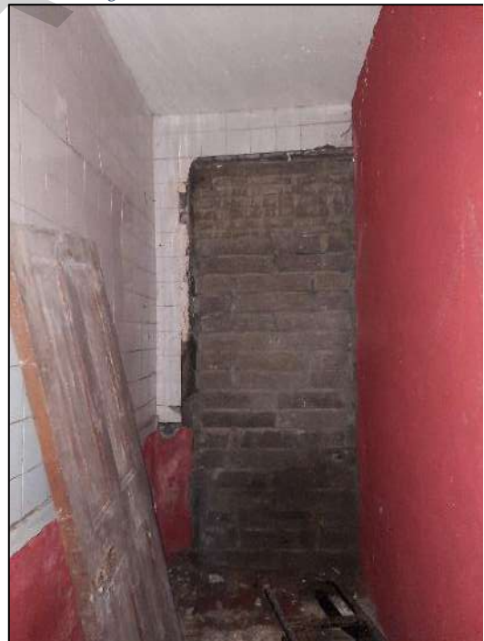
Plate 3-12 Blocked door to the west of the structure.
