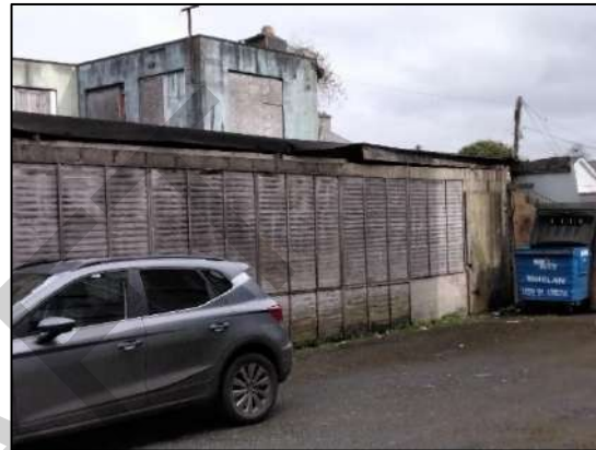
Plate 3-4 Rear structure with access door on right.
