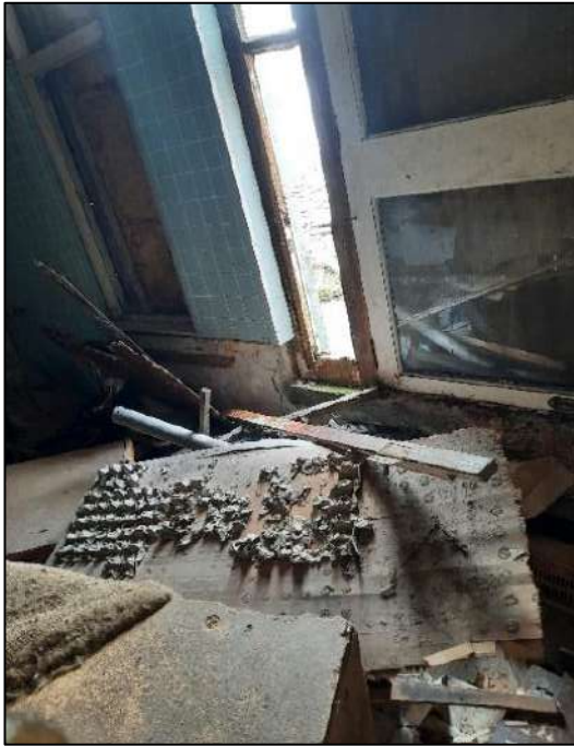
Plate 3-13 1st Floor room to the rear with open external access.
