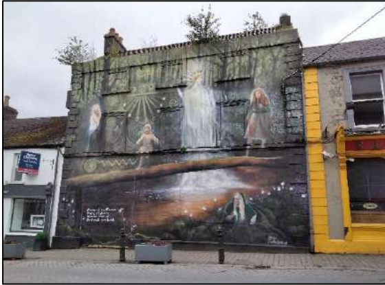
Plate 3-1 Exterior front view of the derelict structure.
