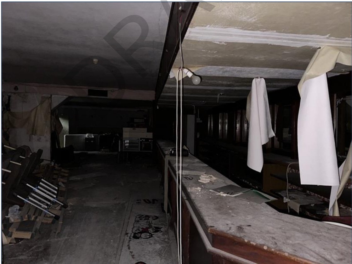
Plate 2-2 Inside of the derelict building at 102 Main Street, Portlaoise.
