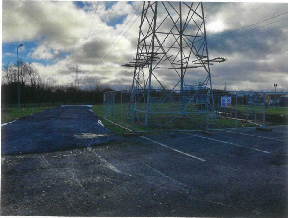
Figure 5 -Typical Heras type Fencing around tower structures.
