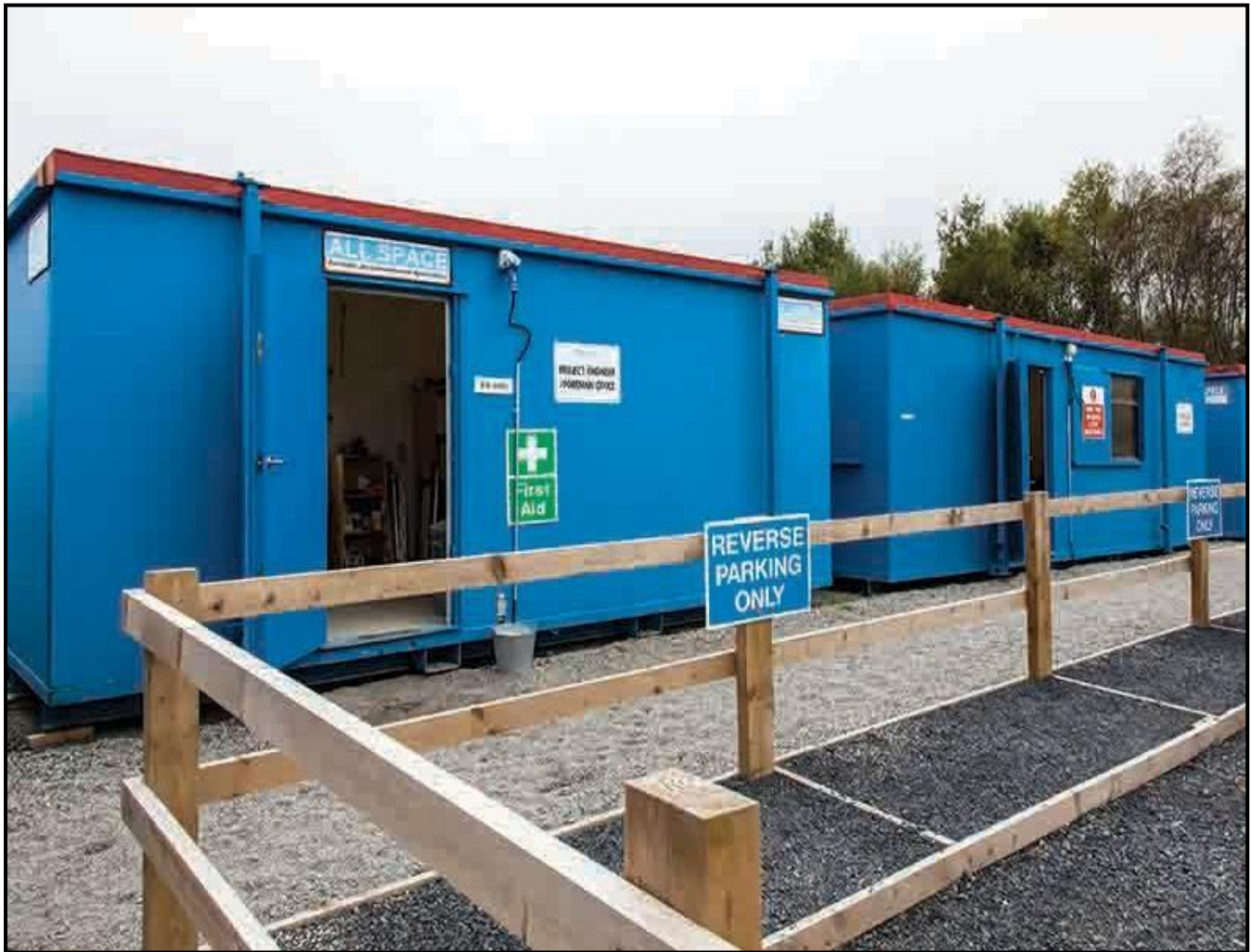
Figure 3: Typical temporary site construction compound
