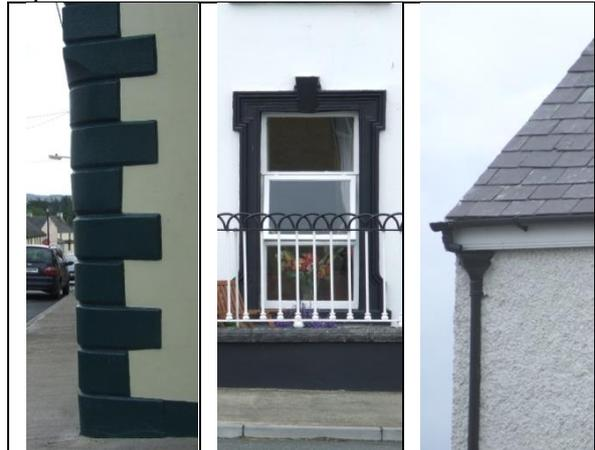
*Building features: chamfered, faux quoins; raised plasterwork window surround with keystone detail and wrought iron railings to front; natural slate roof and cast iron hopper*
