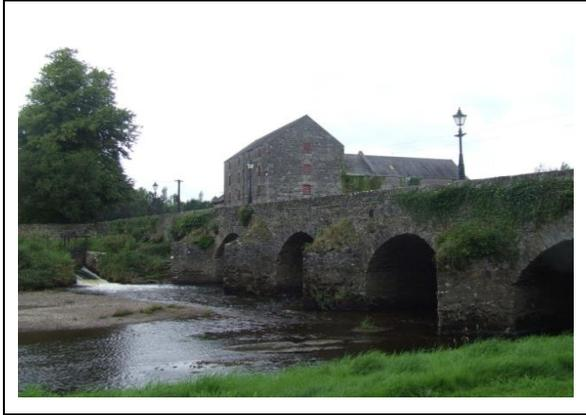
The double row of trees and the six-arch limestone bridge (1750) with rubble stone parapets provides a fitting entrance to the village and can be appreciated from the grassed river banks below. The village has a tidy and well-maintained feel.
