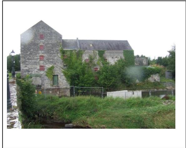
The Corn Mill (1840) (above) of coursed limestone rubble, dressed in brick with limestone quoins, slate roof, red ridge tiles and cast iron rainwater goods is a landmark building. As suggested by its location adjacent to the River, it was water-powered and the mill race, weir and steps along the southern side of the river bank are extant. The bridge spanning the river is sizable and can be appreciated from the banks, it is ornamented by cast iron lanterns. The mill structure is now vacant.
