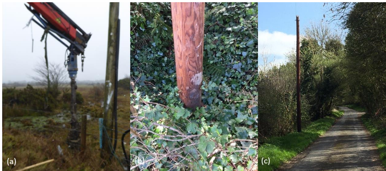
FIGURE 3. (A) UTILITY TRUCK MOUNTED AUGER EXCAVATING HOLE FOR UTILITY POLE, (B) AND (C) NEWLY INSTALLED UTILITY POLES.
