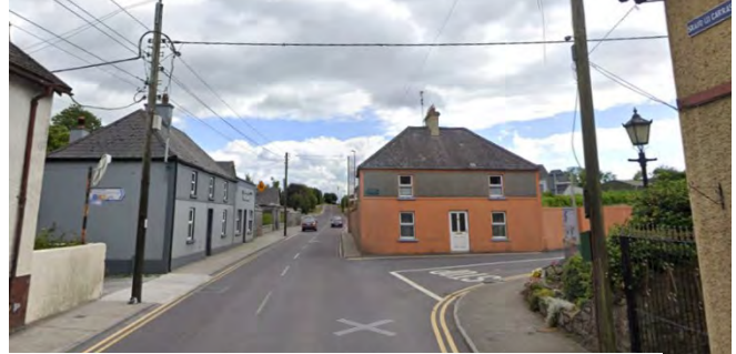
Fig.3 Existing dwelling at corner of site
