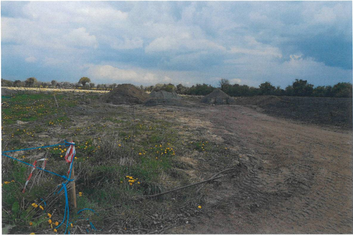
Photo 1: Stockpile of excavated soil
