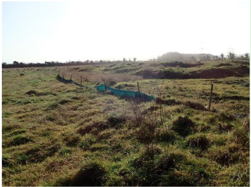
Plate 6 – silt fencing around spoil areas
