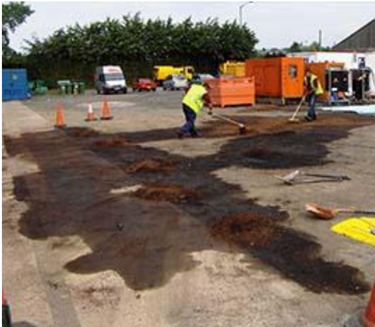
Figure 4: Showing spill clean up using spill kits
