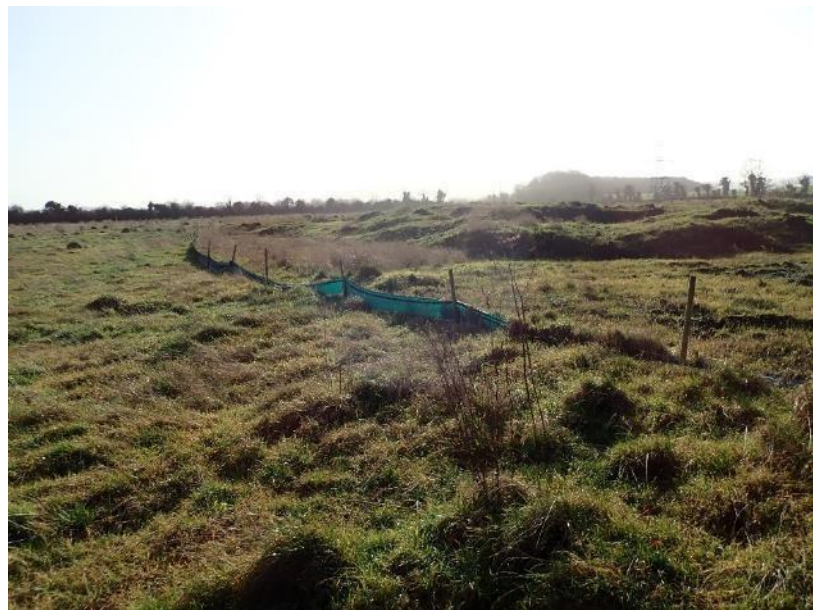
Plate 6 – silt fencing around spoil areas
