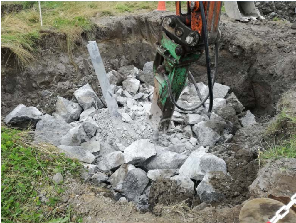
Photograph 5 Tower leg removal.
