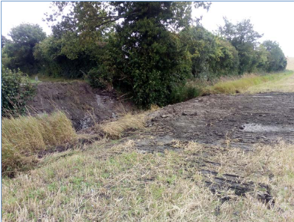
Photograph 11 Reinstated Drain and Dry Bank following removal of drain crossing.
