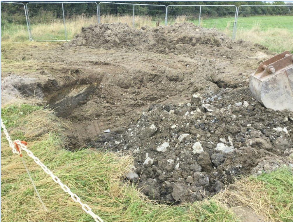
Photograph 9 Tower leg reinstatement with subsoil.
