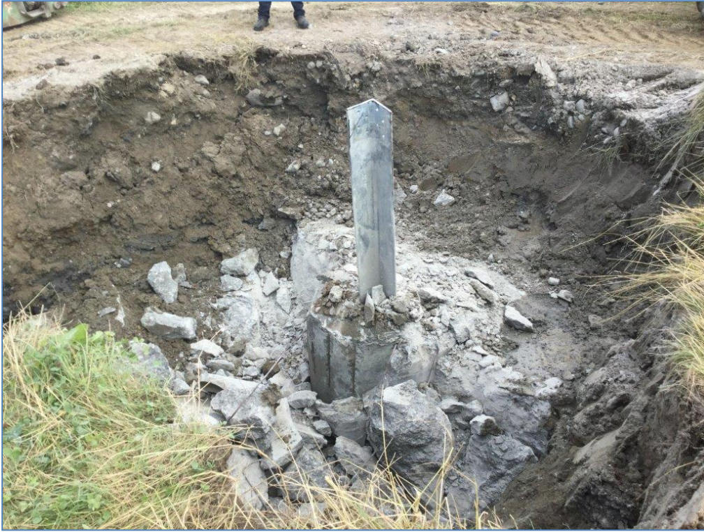
Photograph 6 Tower leg removal.
