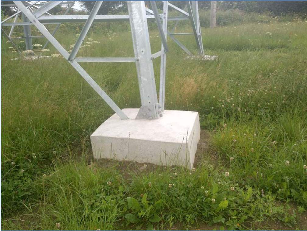
Photograph 4 Tower legs pre-removal.
