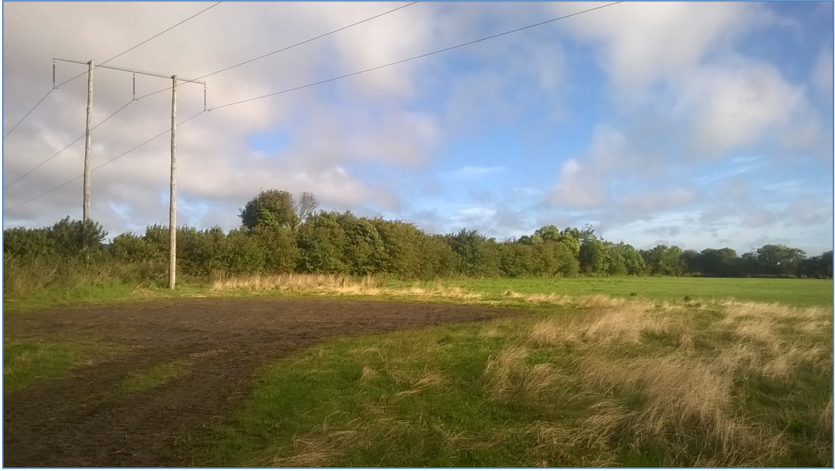
Photograph 10 Site location following restoration works.
