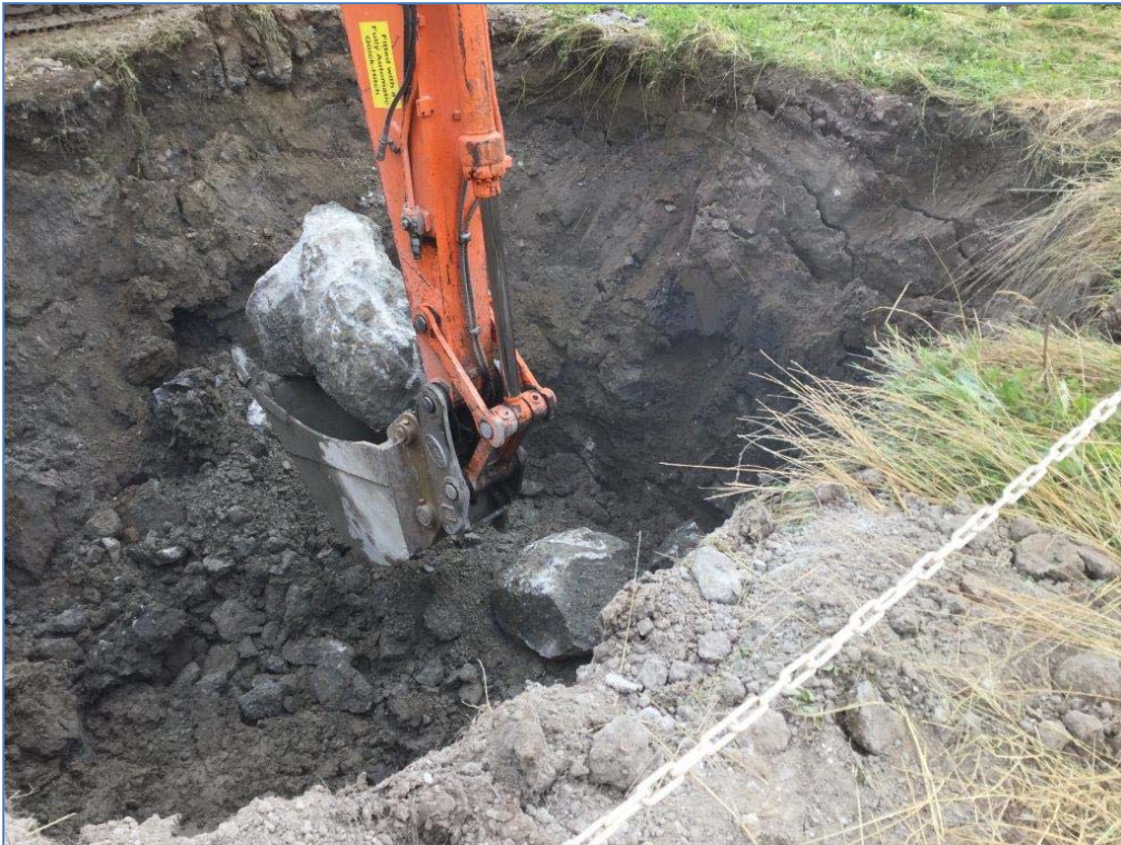
Photograph 7 Tower leg removal.
