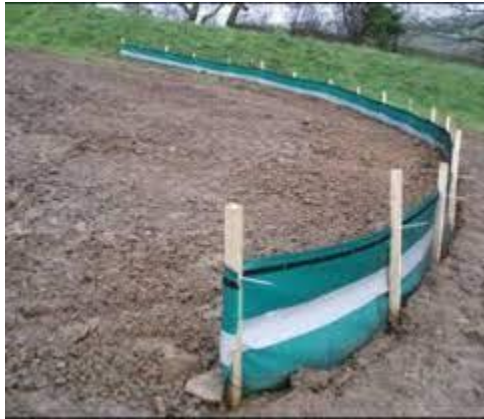
Figure 02 - Example of Silt Fencing
