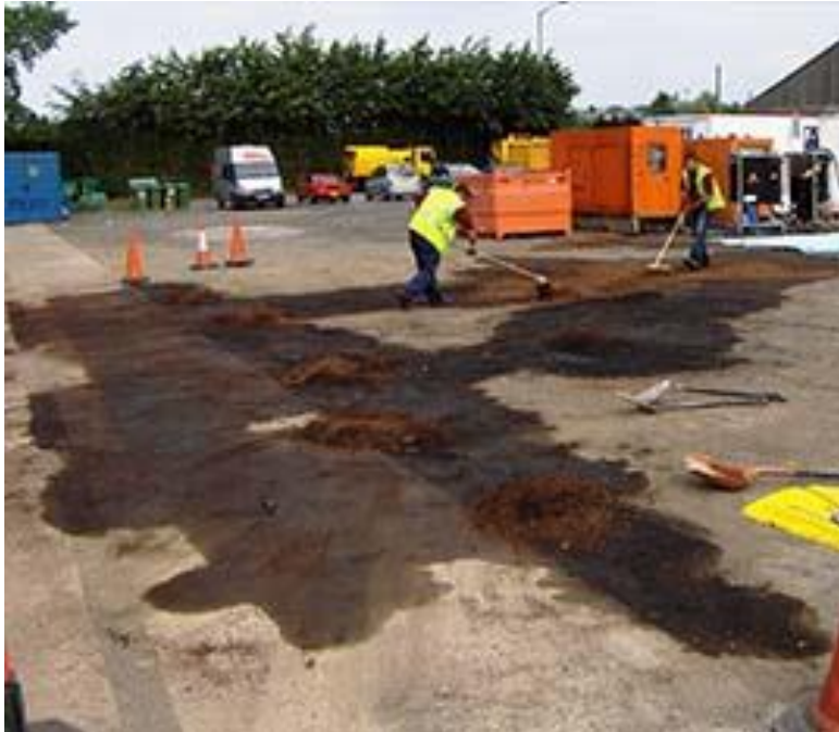
Figure 4: Showing spill clean up using spill kits
