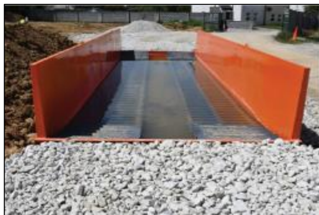
Figure 18: Stone access ramps in place
