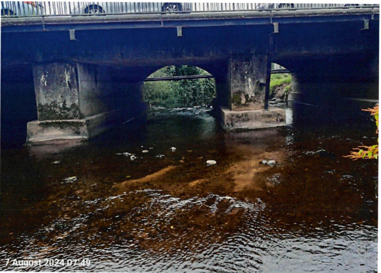
Covent Bridge, After
