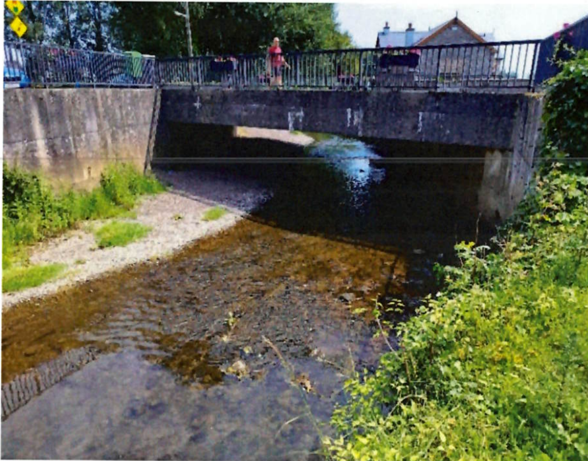
Irishtown Bridge, Before
