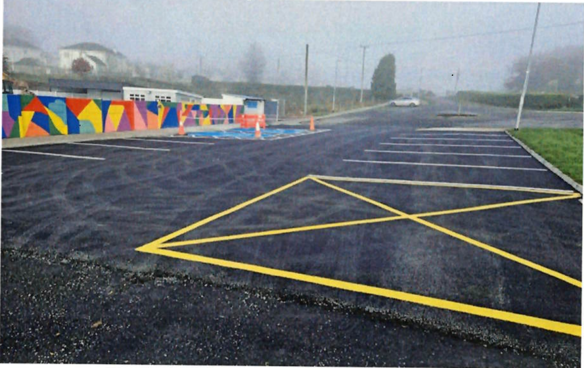
Carpark Surfacing, Ballinakill Swimming Pool
