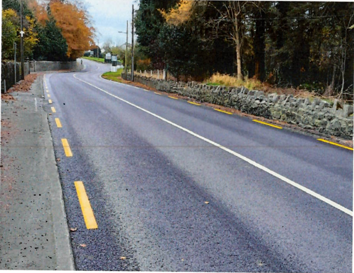
Road resurfacing R430 Carlow Road Abbeyleix
