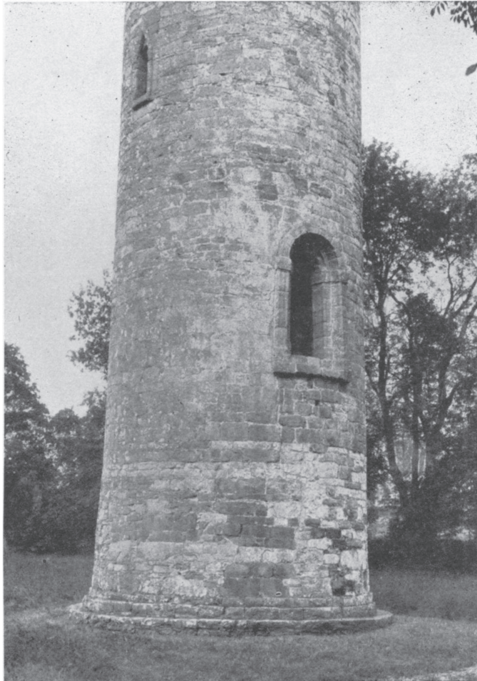
TIMAHOE ROUND TOWER. (The Lower Part, showing the doorway, window, and footings.)
