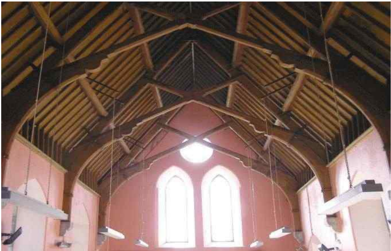
Figure 20: Interior of former church
