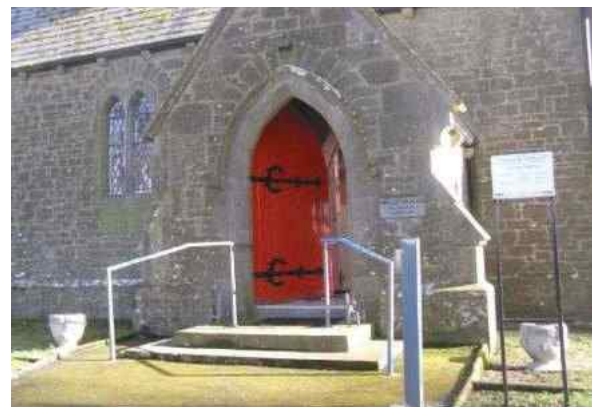
Figure 19: Stepped access to church
