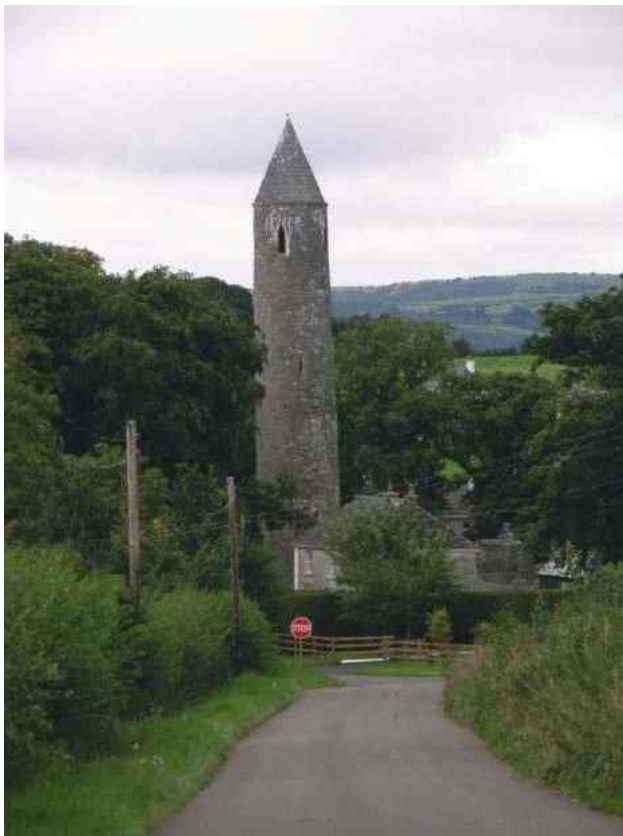
Figure 22: View of tower when approaching along the Pike Road.
