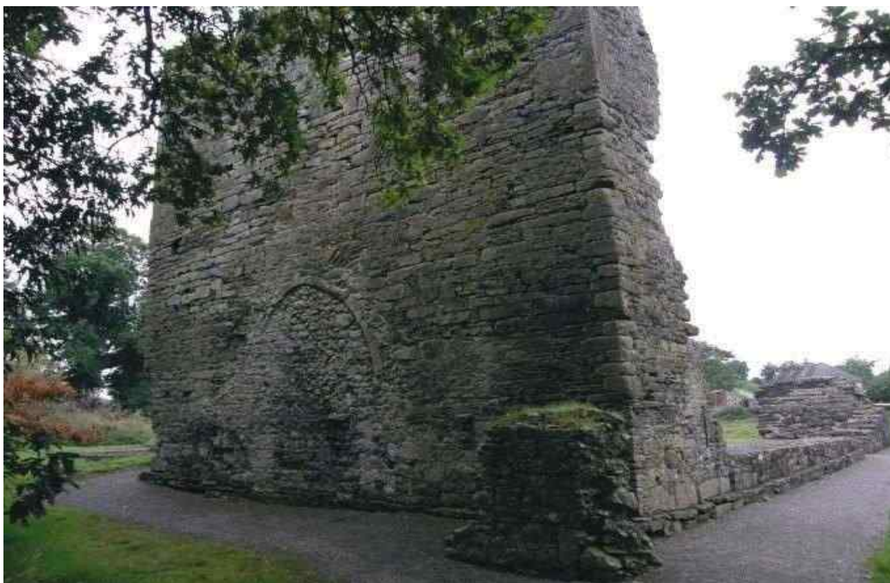
Figure 8: Gable of church/castle with blocked arch
