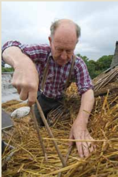
Michael Dempsey places a hairpin scollop into position, before hammering it in to hold the straight scollop that will secure a fresh layer of thatch.
