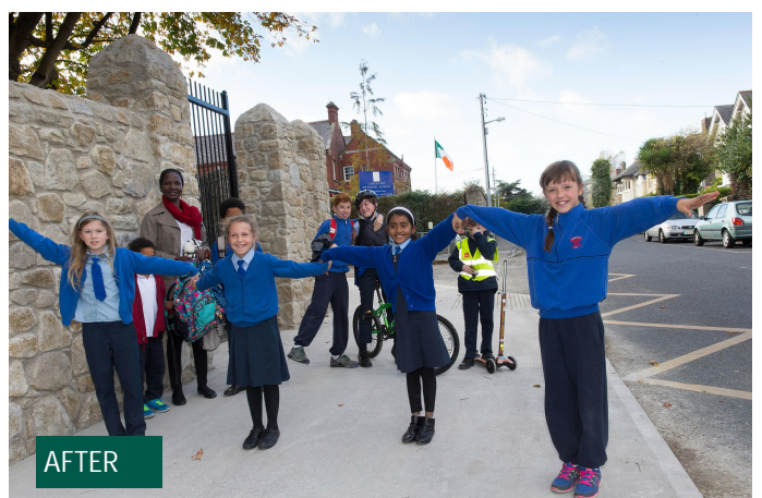
New widened footpath (Photo: DLRCC)
