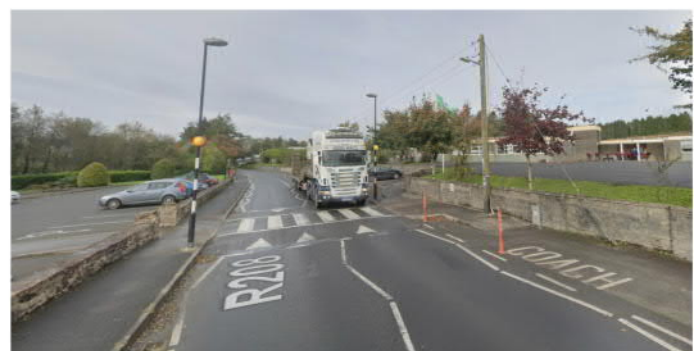
New raised zebra crossing at school entrance (Image: Google Street View)
