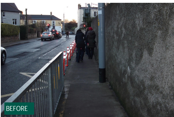
Narrow footpath on Convent Road (Photo: DLRCC)
