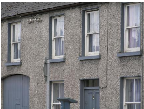
Fig 20. Historic sash windows with original glass on Grattan Street.
