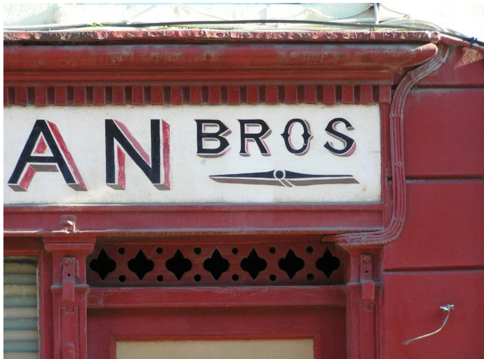
Fig 21. Detail of Whelan Bros historic shopfront on Main Street
