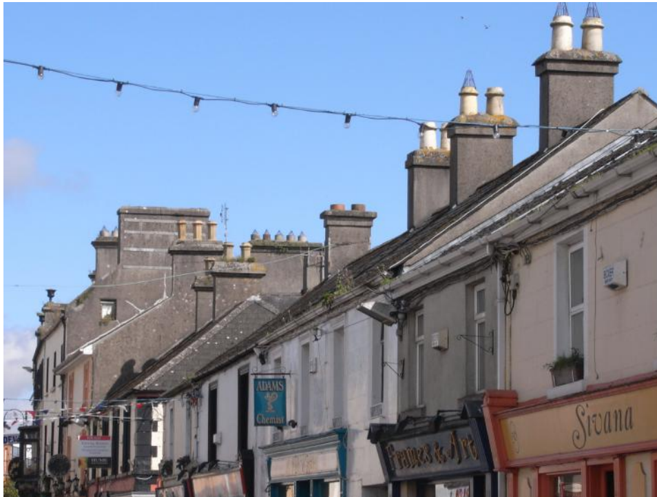
Fig. 23: Roofs along Main Street
