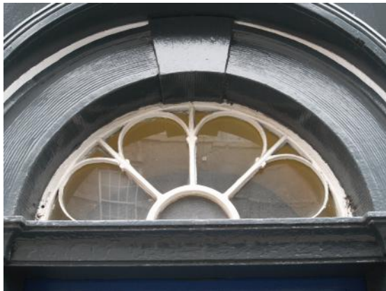
Fig 2. Fanlight on Church Street
