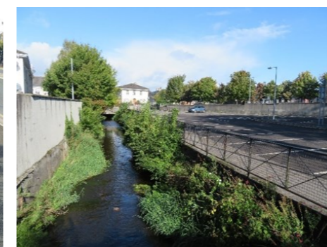
Triogue River, west of Millview Car Park - canalised
