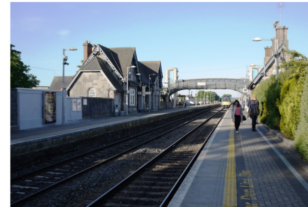
Portlaoise Railway Station
