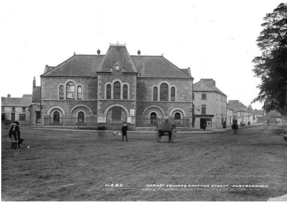
Market House/Town Market Square (Lawrence Collection, c. 1900)
