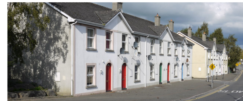
Existing Residences at Church Street
