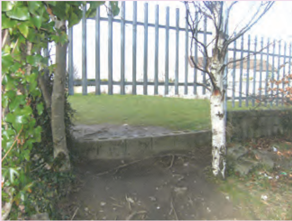
Figure 6.6: Palisade fence at eastern boundary of Dargle Wood, Knocklyon
