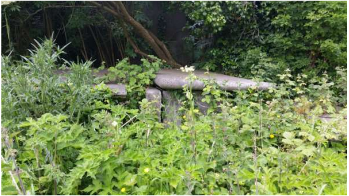
Plate 29: Overgrown box tombs in NW corner of graveyard close to Church tower
