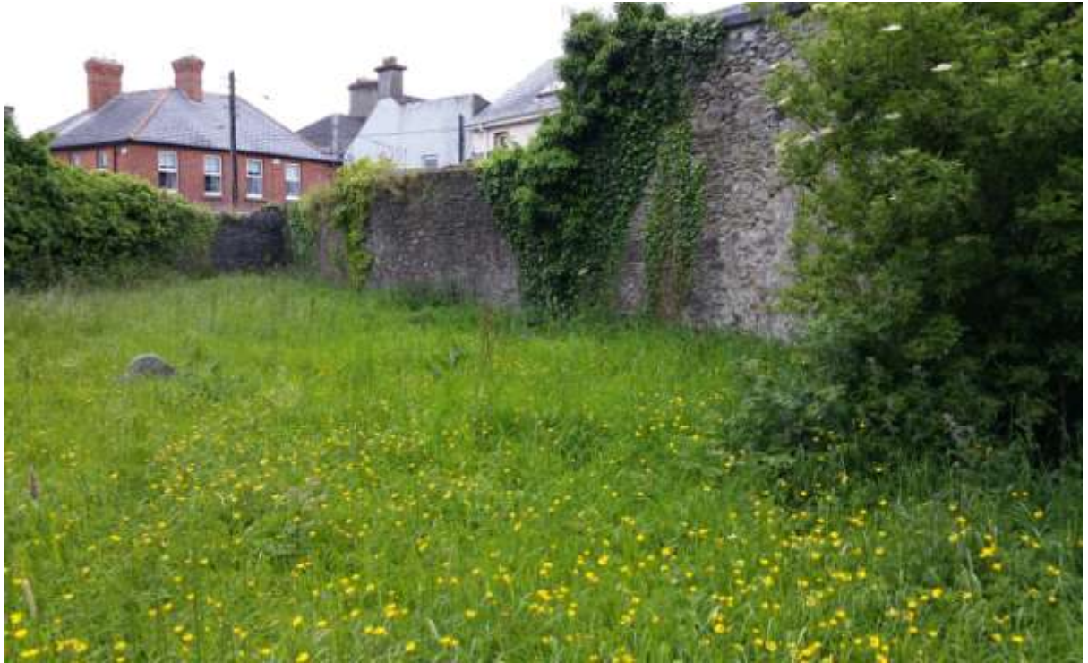
Plate 3: East end of south wall – looking E
