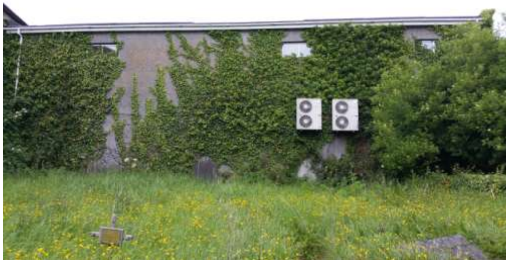
Plate 20: Modern building forming western boundary to site
