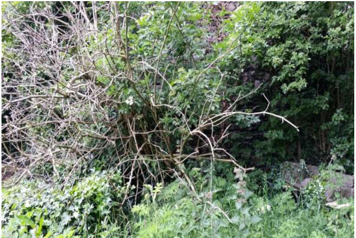
Plate 16: Dense vegetation in NW corner of graveyard close to Church tower
