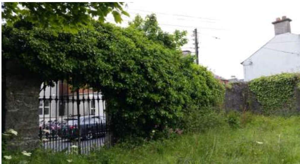
Plate 10: Ivy-clad E wall of graveyard overhanging entrance gates
