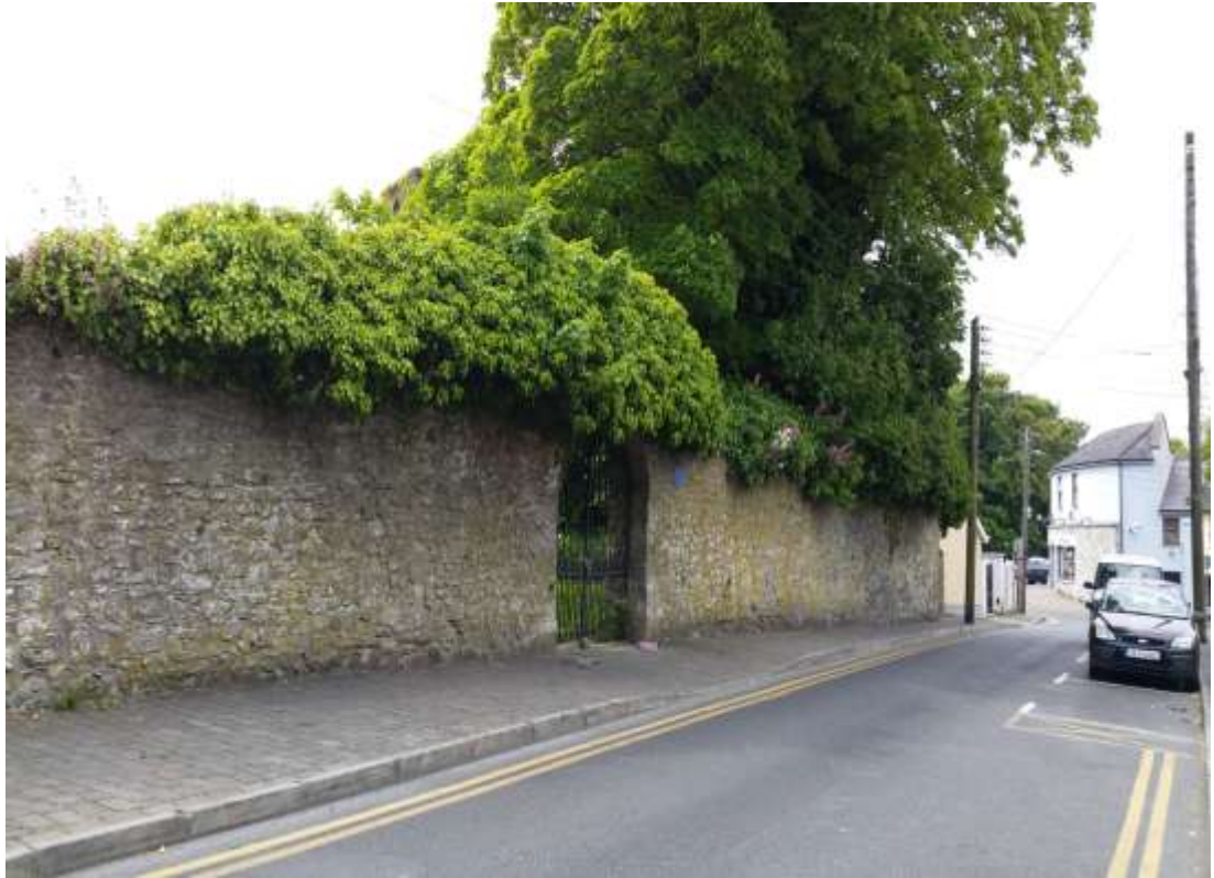
Plate 1: East wall of graveyard and entrance gates – looking NNW
