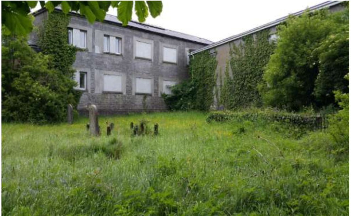
Plate 5: Later buildings forming southwest corner of graveyard
