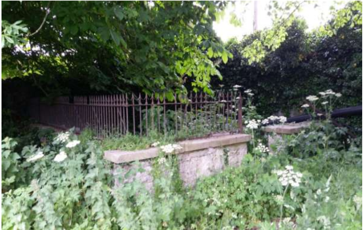
Plate 33: Wall and metal railing surrounding family grave
