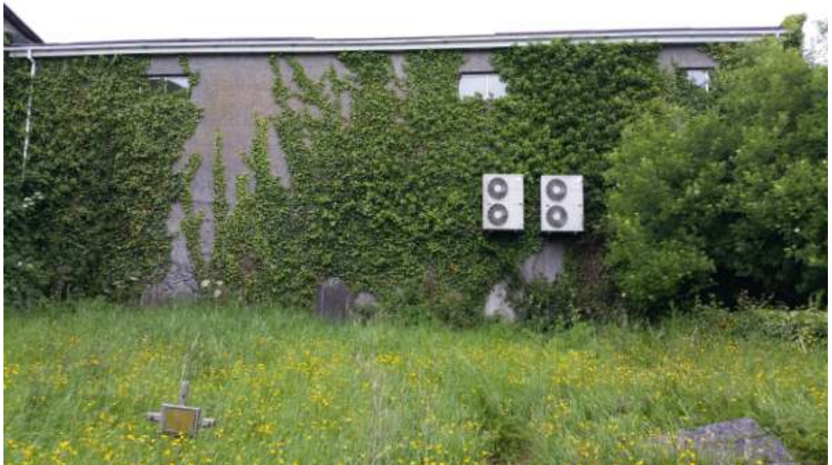
Plate 6: Later building fronting onto Church Street forming southern end of western boundary to graveyard
