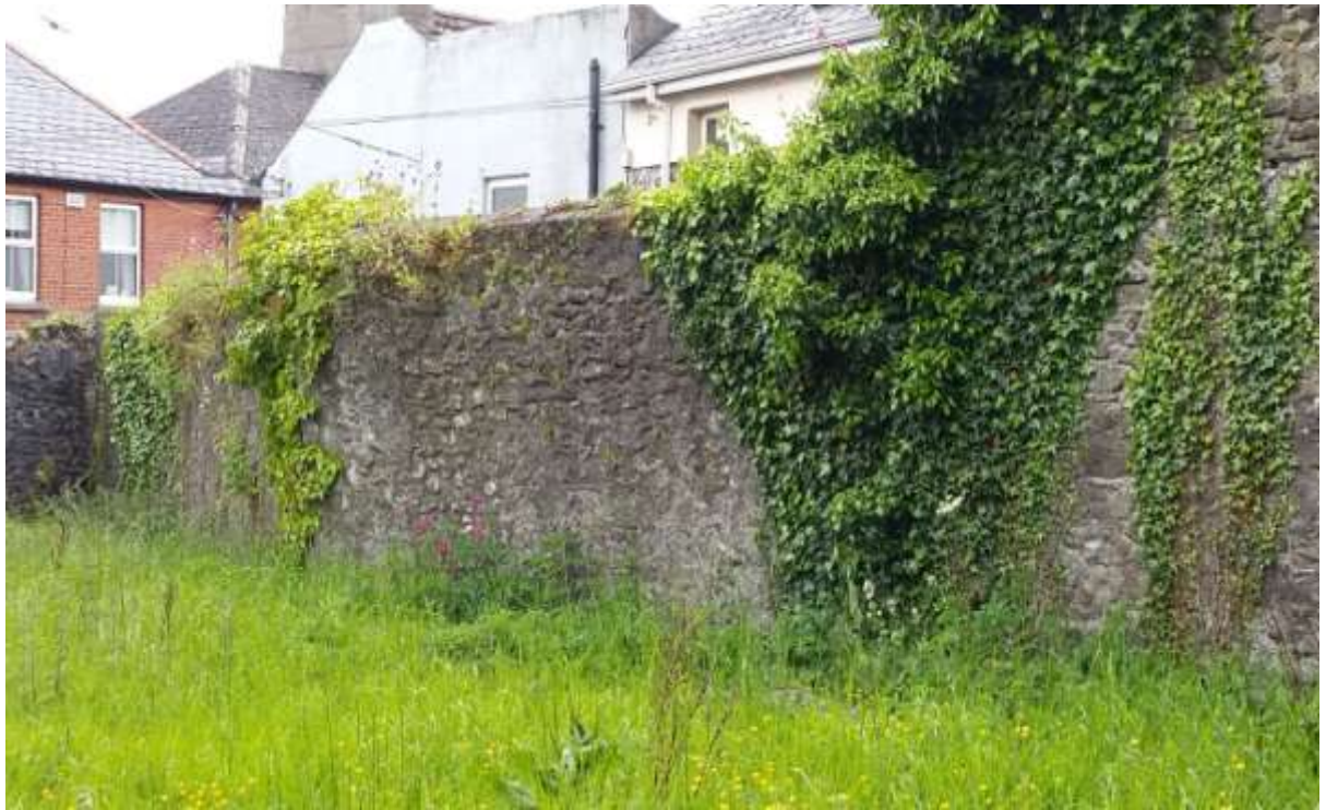
Plate 11: E end of ivy-clad south wall
