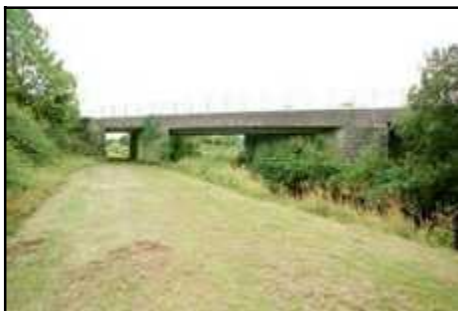
F003_03 22/08/2006 North-west elevation of rail bridge.
