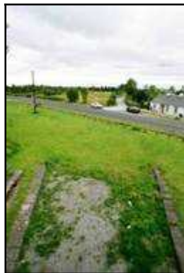
Left: S201_05 Looking north-east along infilled canal from Blackhall Bridge (feature 206).
