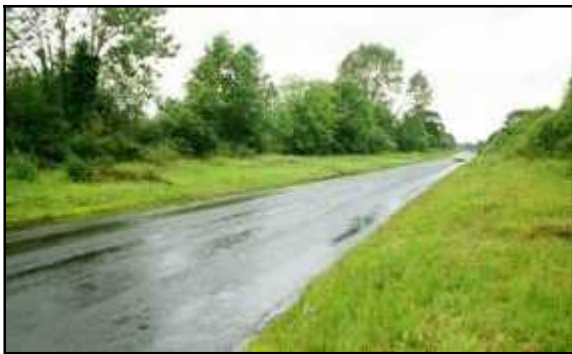
S201_04 Looking west from site of Ballymorris Bridge (feature 204).
