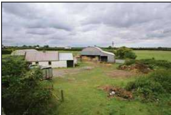
S109_01 Looking north along infilled section from Bergin's Bridge (feature 105).
