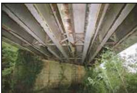
F003_04 22/08/2006 Underside of main span showing RSJs.
