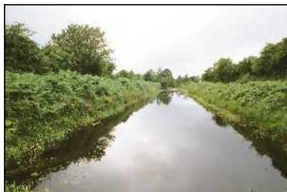
S005_01 Looking NW along section 005 from impounding dam at SE end.
