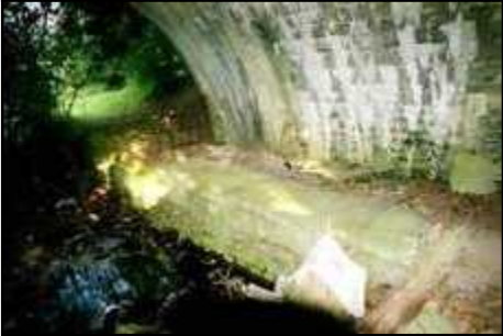
F305_03 14/06/2006 Towpath underneath Dangans Bridge.
