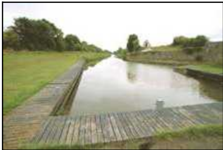
F901_03 22/08/2006 Looking south-west along Grand Canal from bridge (feature 901d).
