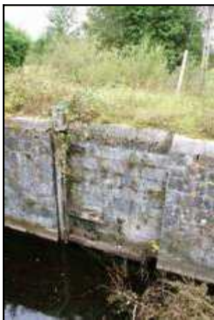
F101a_03 22/08/2006 Gate detail at south-west end of lock chamber.
