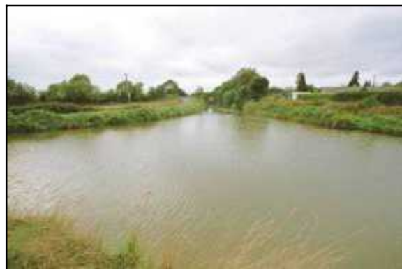
S001_01 Looking north-west across canal junction to first section of Mountmellick Canal.
