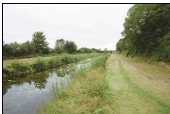
S003_01 Looking north-west from road bridge (feature 001).
