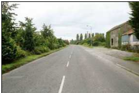
S201_01 Looking south-west from lock (feature 201a).
