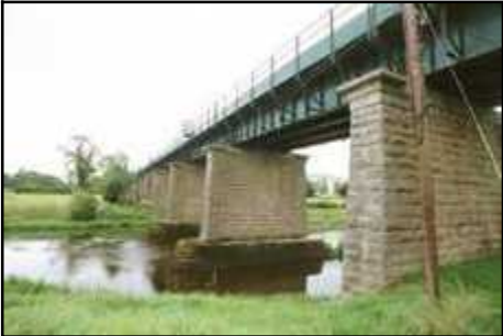
F902_02 22/08/2006 Pier detail at west end of Barrow Bridge.
