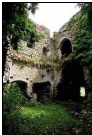
F910_02 22/08/2006 East section, from north-west.
