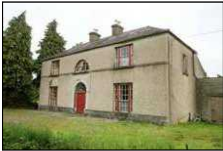
F923_02 22/08/2006 Front door detail.
