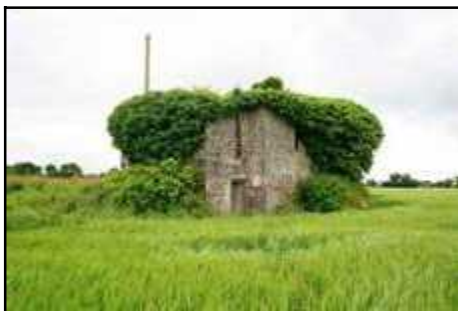
F301c_03 29/06/2006 NE bay of house (kitchen), looking south.
