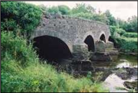
F928_02 17/06/2004 South (upstream) elevation, from left bank.
