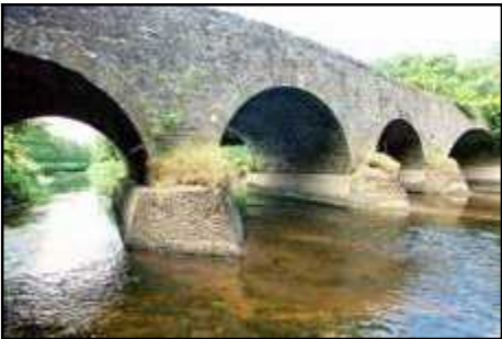
F928_03 17/06/2004 North (downstream) elevation, from right bank.
