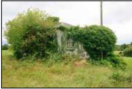
F301c_02 29/06/2006 Lock house from north.
