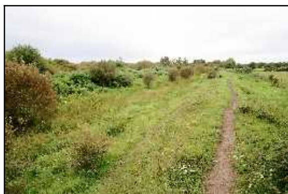
S102_02 Looking north-west along dewatered canal from just north of lock 1 (feature 101a).
