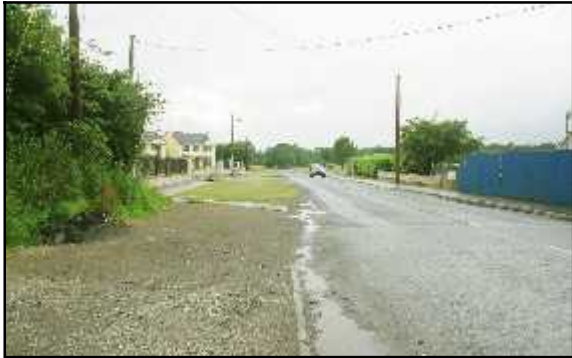
S201_03 Looking west from Odlum's Mill (feature 914).
