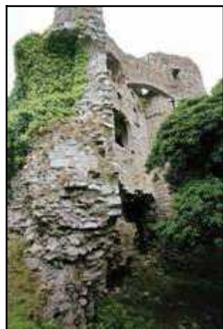
F910_03 22/08/2006 East elevation of west section, from south-east.
