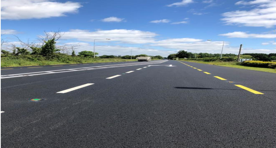
Resurfacing Works Completed on R445 (Former N7) - View Towards Monasterevin
