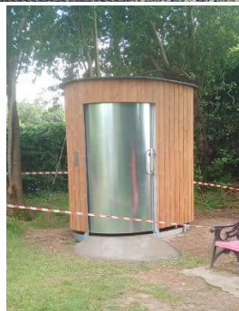
Images of some of the new equipment & accessible toilet – Ballylinan Playground
