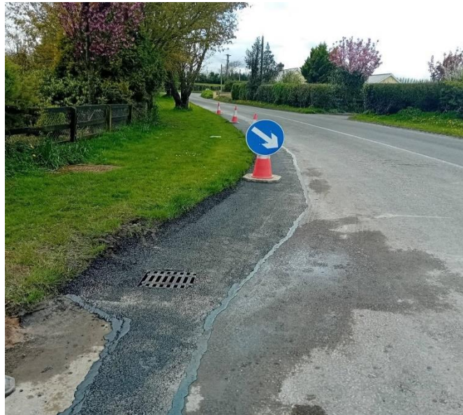
Drainage works, Ross
