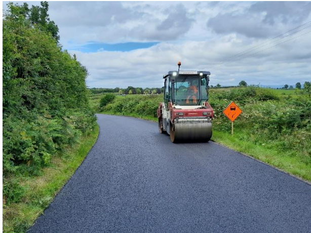
Road strengthening works at Clonreher & Tullore
