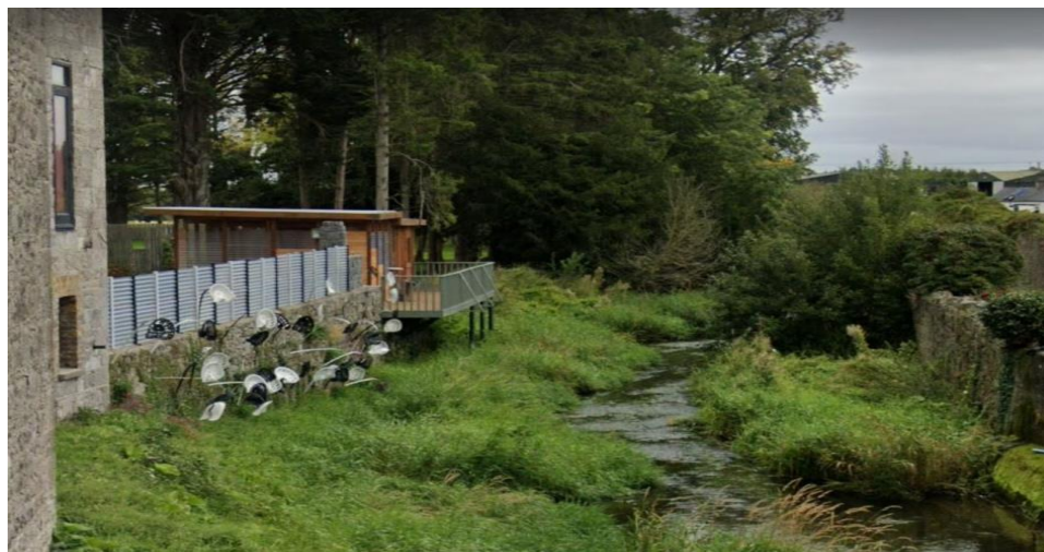
Stradbally River at N80 Bridge, Stradbally - Before Silt Removal Works Commenced
