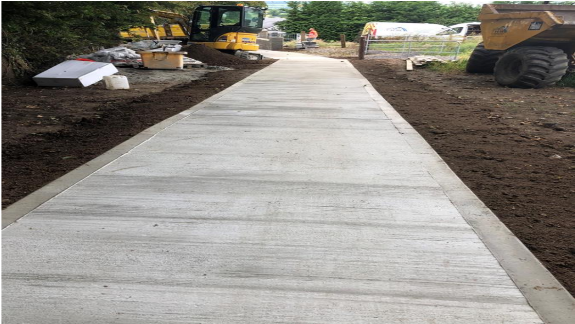
New Footpath for National School - Works in Progress August 2024
