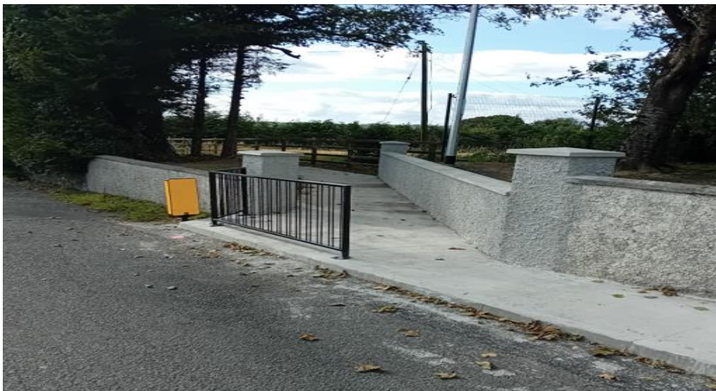
New Footpath for National School - September 2024
