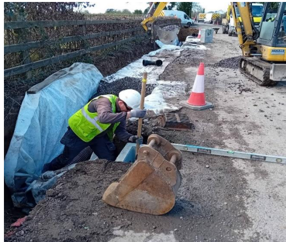
Drainage works, Clonreher
