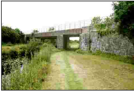
F003_01 22/08/2006 South-east elevation of rail bridge.
