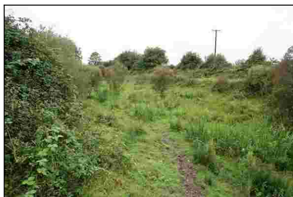
S102_01 Looking north-west along dewatered canal from just north of lock 1 (feature 101a).
