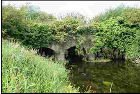
F309_02 14/06/2006 Mountmellick Aqueduct from upstream (south) side.
