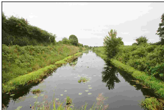
S003_02 Looking south-east from impounding dam at NW end.
