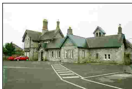
F916a_01 29/06/2006 Station building (north), from north-west.
