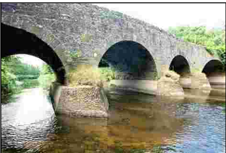
F928_03 17/06/2004 North (downstream) elevation, from right bank.
