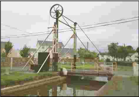
F901a_02 22/08/2006 Draw bridge, from west.
