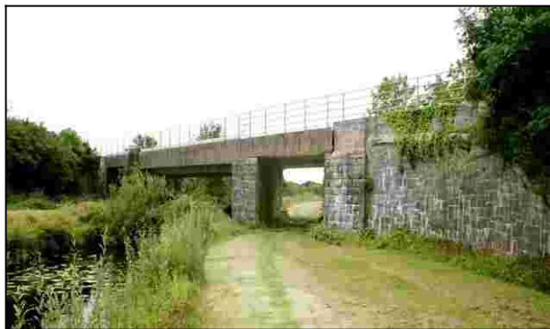
Fig 5.5a Railway bridge west of Monasterevin.
