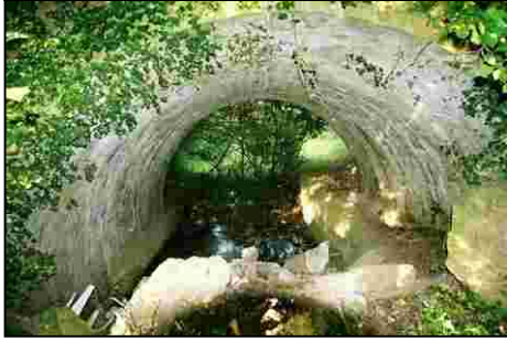
F305_02 14/06/2006 Dangans Bridge: inside of arch, from west.
