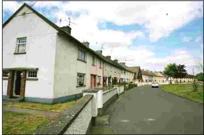
Fig 6.9 Council houses at Mountmellick.
