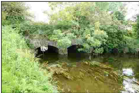
F309_03 14/06/2006 Mountmellick Aqueduct from downstream (north) side.
