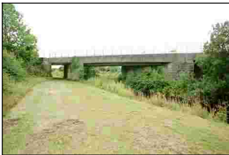
F003_03 22/08/2006 North-west elevation of rail bridge.
