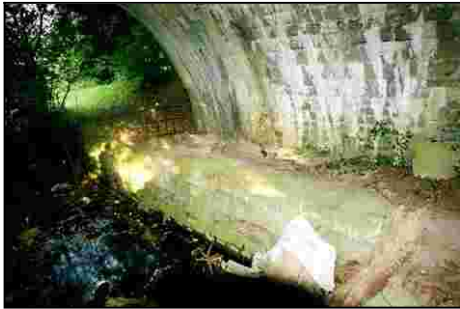
F305_03 14/06/2006 Towpath underneath Dangans Bridge.
