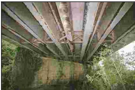
F003_04 22/08/2006 Underside of main span showing RSJs.
