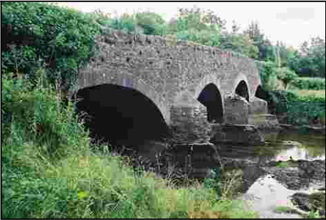
F928_02 17/06/2004 South (upstream) elevation, from left bank.
