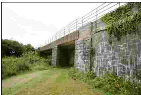
F003_02 22/08/2006 South-east elevation of rail bridge.
