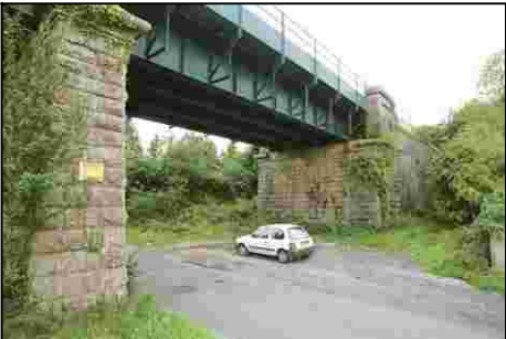
F902_03 22/08/2006 Abutment detail at west end of Barrow Bridge.
