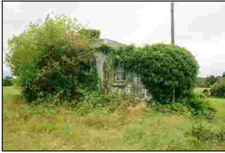
F301c_02 29/06/2006 Lock house from north.
