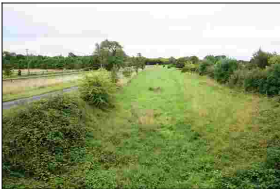
S103_02 Looking east from Wheelahan's Bridge (feature 103) along infilled section.
