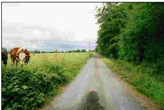
S203_01 Looking north-east along line of road towards Woodbrook Bridge (feature 207).
