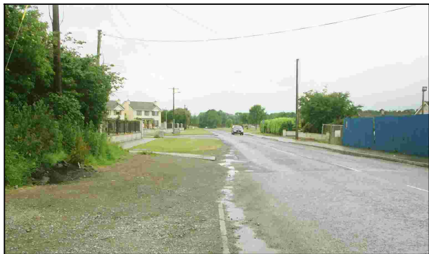
Fig 3.2c Reach 2 – Portarlinton ring road, west of Odlum’s Mill.
