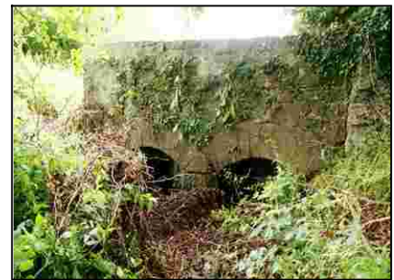
Fig 5.6 Culvert at Kilbride.
