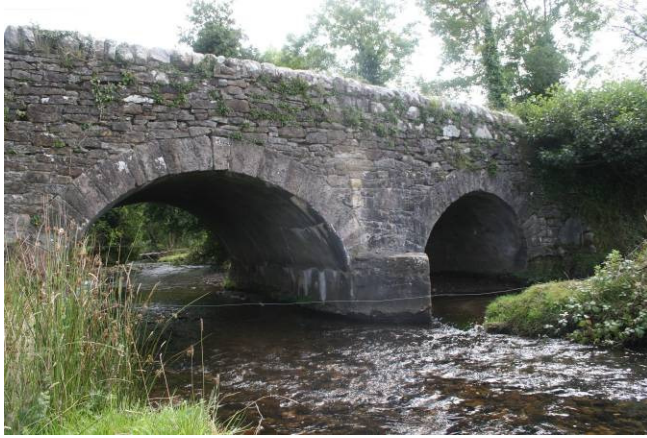
Pluck's Bridge (upstream)
