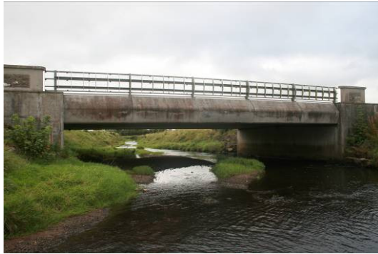
Ballyclare Bridge (upstream)
