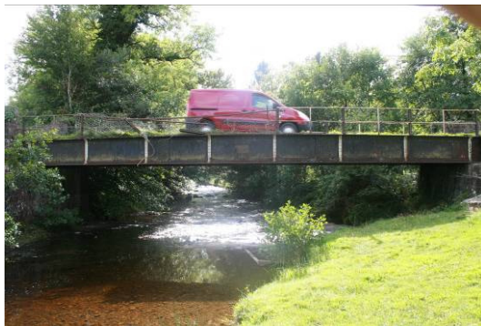
Lacca Bridge (upstream)
