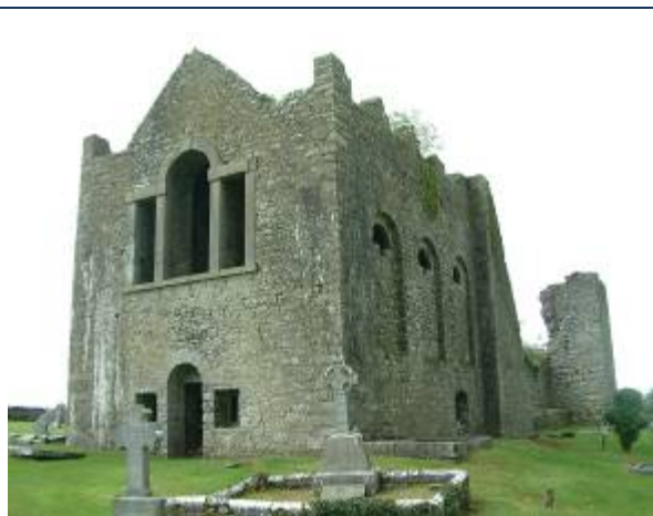
Chancel mortuary and nave, looking south-west
