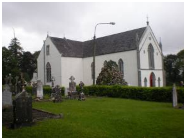
General view of the site and St. Lazerian's Church, facing northwest
