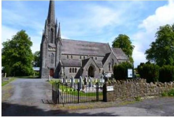
Overview of the burial ground and Church of Michael & All Angels, looking north
