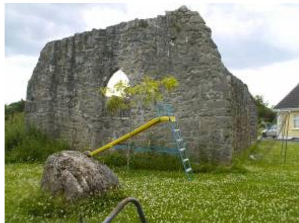
Eastern gable of church, looking west
