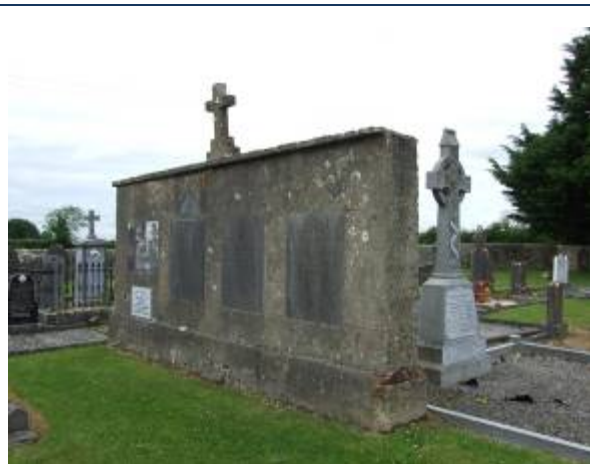
Retention of wall of 18 th century church, facing northwest
