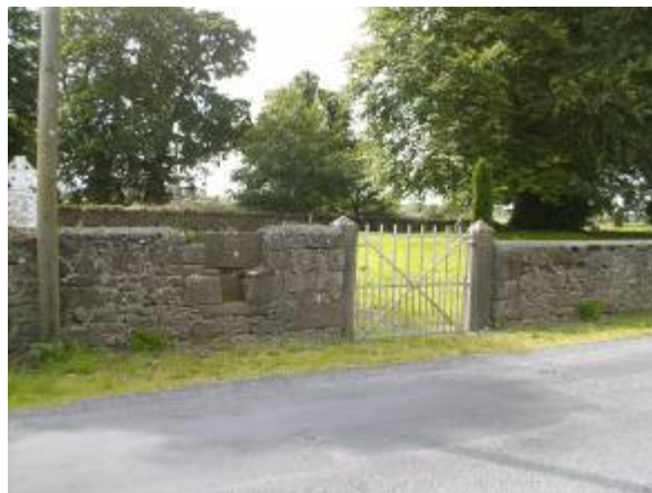
Wrought iron gate and stone stile in eastern boundary wall, looking northwest
