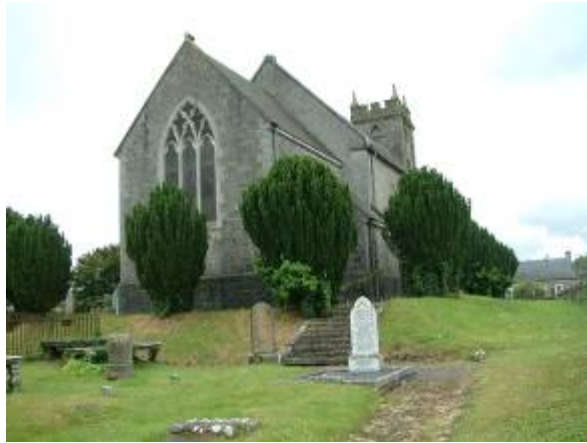
The church is itself elevated above the burial ground which is raised above the surrounding ground to the north and west, looking south-west
