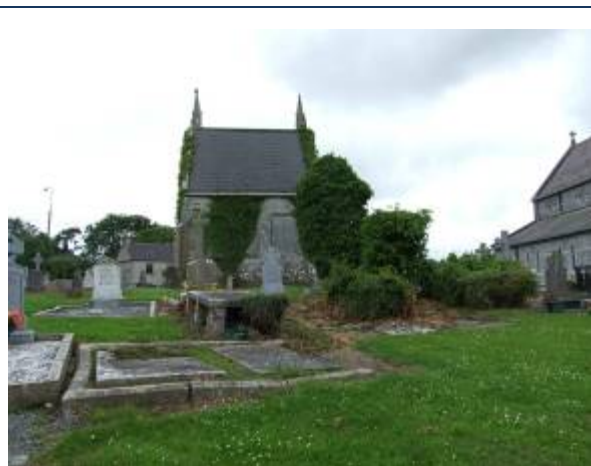
View of the Grace Mausoleum, facing west
