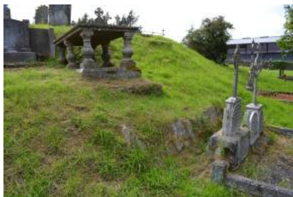
The huge mound at Clonenagh with precariously placed memorials, looking northwest
