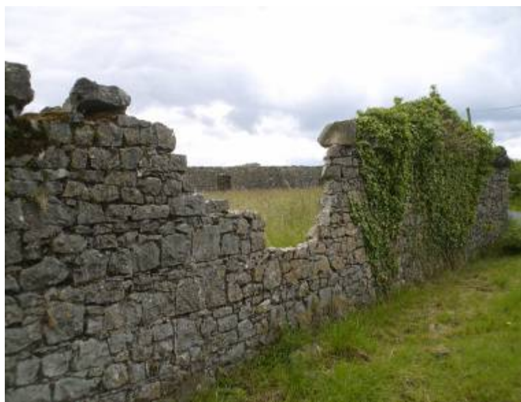
Northern boundary wall of burial ground, looking south towards church ruins
