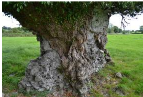
Ivy has been allowed to grow to the extent that complete removal would risk structural collapse
