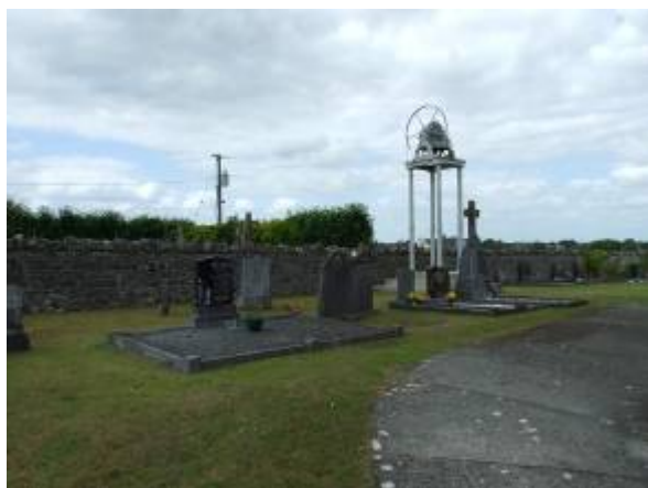
View of the site and bell-tower, facing northwest
