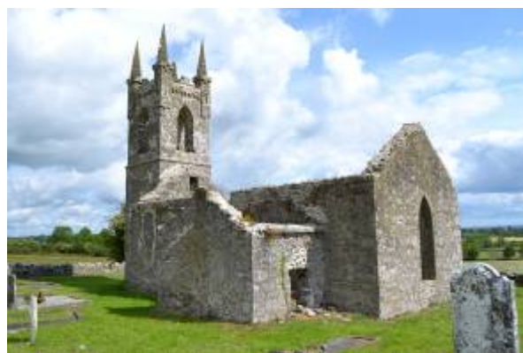
Overview of the restored ruins, looking north
