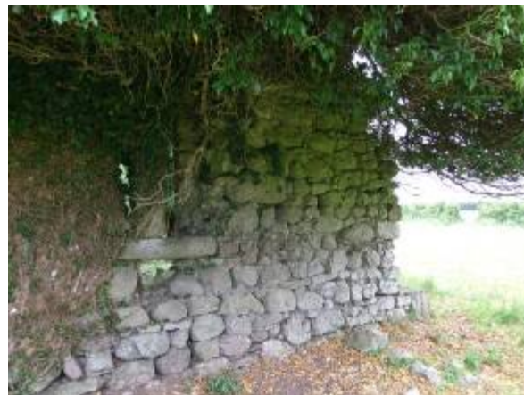
View of the eastern gable of the church ruins, facing south
