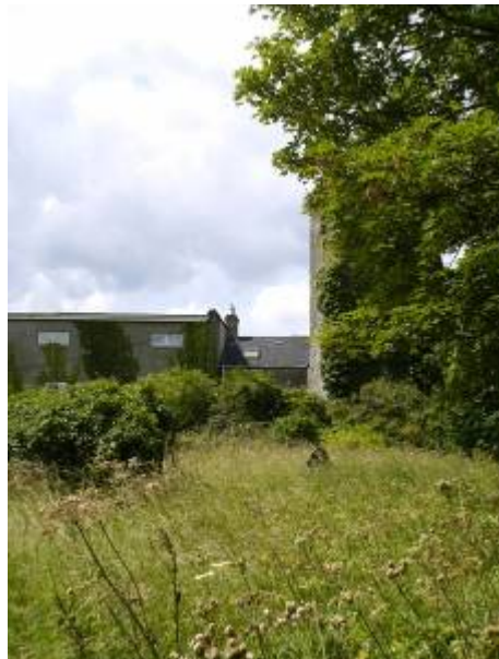
View through the gate of the church tower in the northwest corner, looking west
