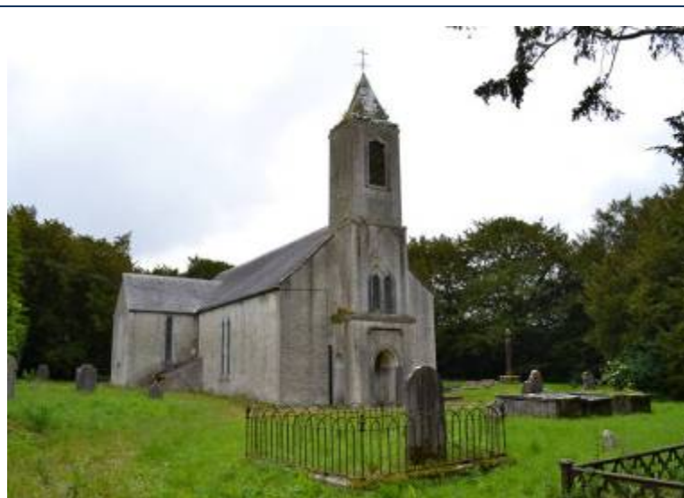
Overview of burial ground and church, looking south.
