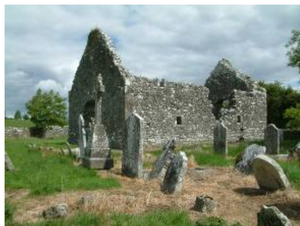
View of church across burial ground, looking northeast
