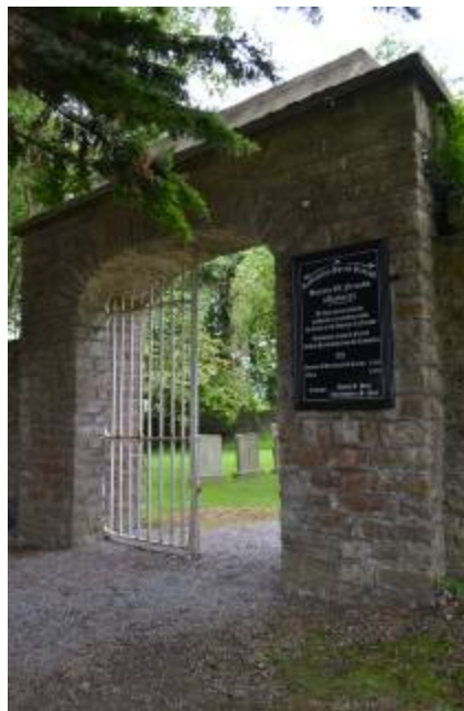
Arched entrance at the Society of Friends burial ground, looking west
