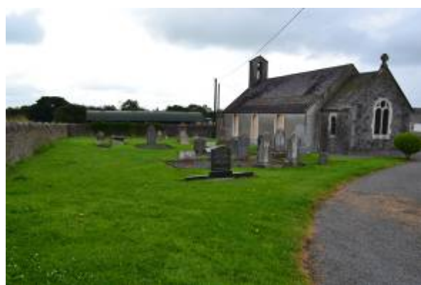
Overview of south side of the burial ground, looking northwest
