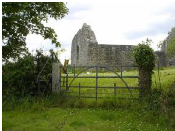
Stone piers, wrought iron gate and stile in north-eastern boundary, looking southwest towards church
