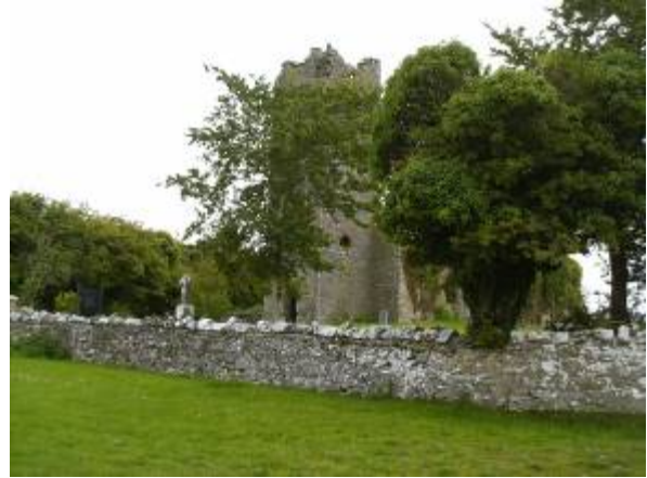
South-western boundary wall, looking north
