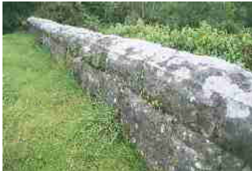
LAIAR-035-010_03 FWH 28/09/2007 Downstream (SW) parapet detail
