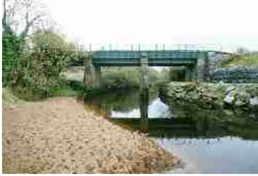
LAIAR-017-030_01 FWH 01/11/2007 Upstream (NW) elevation, from NW.
