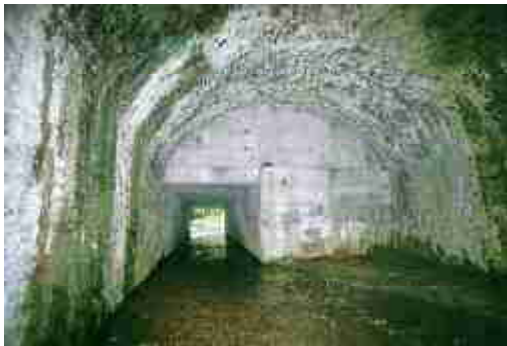
LAIAR-025-017_03 FWH 17/10/2007 Upstream view through arch showing concrete extension.
