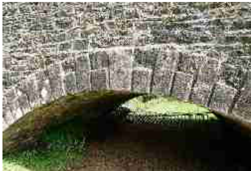
LAIAR-016-006_03 FWH 30/08/2007 Voussoir detailing on upstream/right-bank arch.
