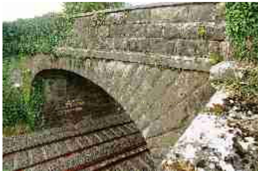
LAIAR-022-017_03 FWH 31/08/2007 Radial spandrel and parapet detailing on SW side.
