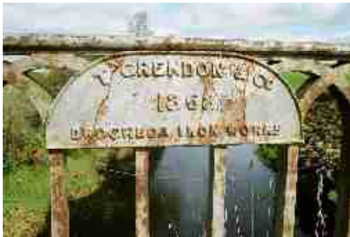
LAIAR-016-013_03 FWH 30/08/2007 Grendon plaque on downstream (east) railing.
