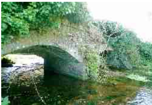
LAIAR-028-010_02 FWH 27/09/2007 Downstream (NE) elevation showing original masonry bridge.
