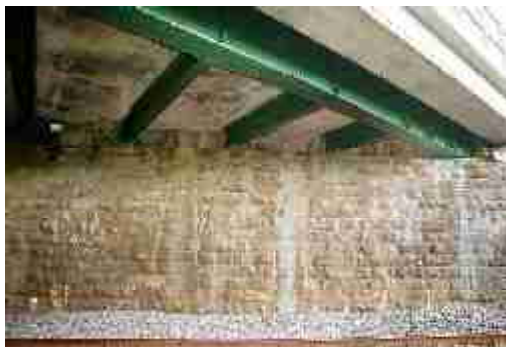
LAIAR-022-016_03 FWH 31/08/2007 Underside of deck.
