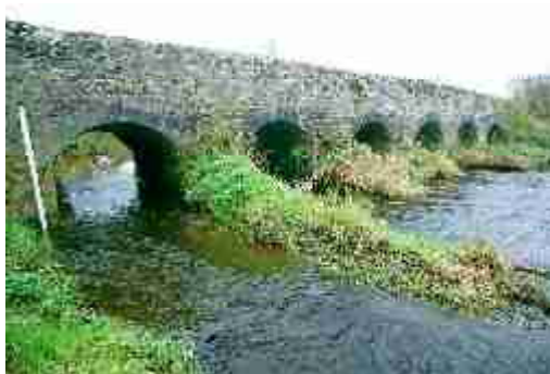
LAIAR-017-033_03 FWH 01/11/2007 Downstream (E) elevation from right bank.
