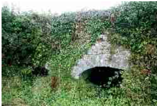
LAIAR-029-012_05 FWH 28/09/2007 Downstream elevation of flood arches on west approach.
