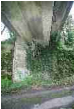
LAIAR-025-023_03 FWH 17/10/2007 Underside of deck.
