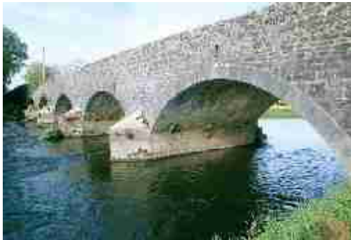
LAIAR-026-006_03 FWH 18/10/2007 Downstream (S) elevation, from SE.
