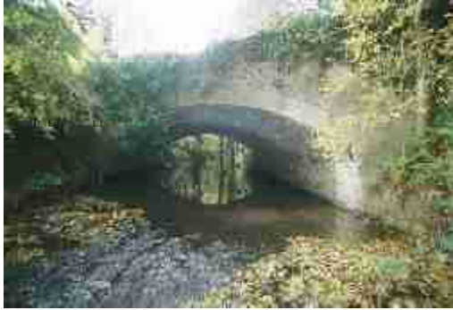
LAIAR-026-011_02 FWH 18/10/2007 Soffit and abutment detail at downstream left-bank end.
