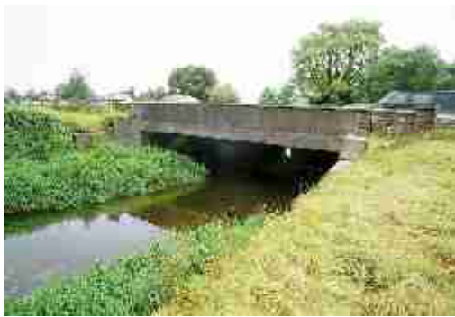
LAIAR-021-008_02 FWH 31/08/2007 Upstream (N) elevation showing 20th century addition.
