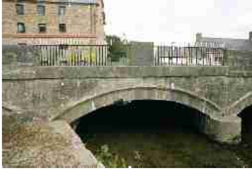
LAIAR-019-021_05 FWH 10/05/2007 Stonework detail on upstream right-bank arch.
