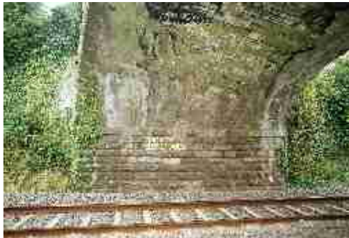
LAIAR-022-017_02 FWH 31/08/2007 Soffit detail. Note skewly laid stonework.
