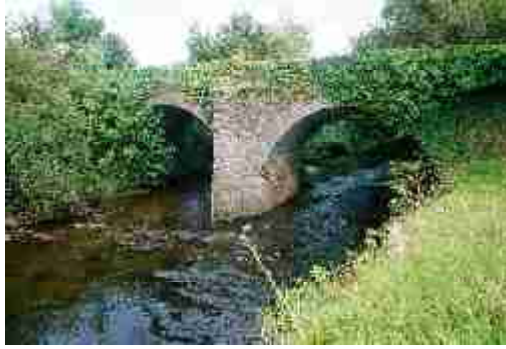
LAIAR-016-005_02 FWH 30/08/2007 Corbel stones on right-bank (south) arch abutment.
