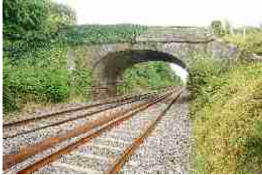
LAIAR-022-017_02 FWH 31/08/2007 Soffit detail. Note skewly laid stonework.
