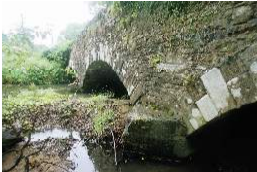
LAIAR-016-003_02 FWH 14/06/2007 Upstream spandrel and cutwater detail.
