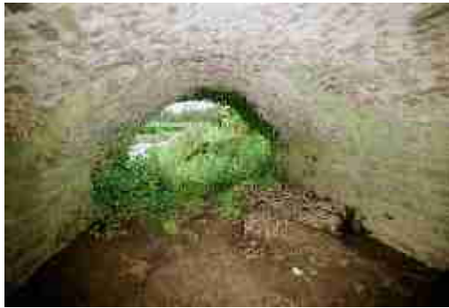
LAIAR-016-015_06 FWH 30/08/2007 Looking up 2nd arch from left bank, showing soffit break. Note arch voussoir.
