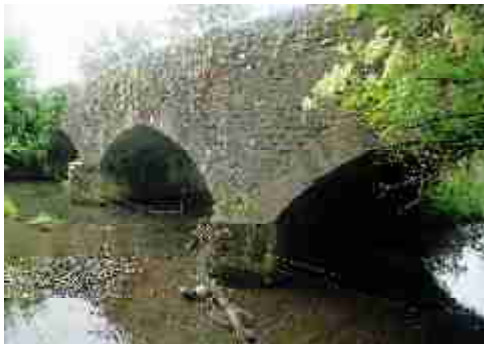
LAIAR-016-002_03 FWH 14/06/2007 Pier and spandrel detail on upstream elevation.
