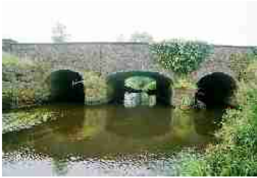
LAIAR-021-008_01 FWH 31/08/2007 Downstream (S) elevation showing original masonry arch bridge.
