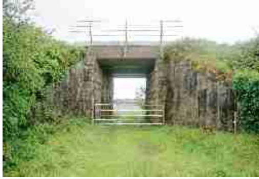
LAIAR-017-020_02 FWH 13/06/2007 Abutment detailing.
