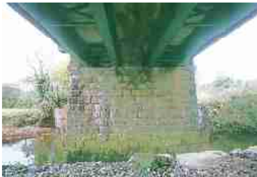
LAIAR-017-030_04 FWH 01/11/2007 Underside of deck (right-bank span).
