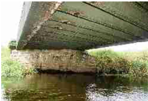
LAIAR-021-005_02 FWH 31/08/2007 Underside of deck and left (W) abutment.
