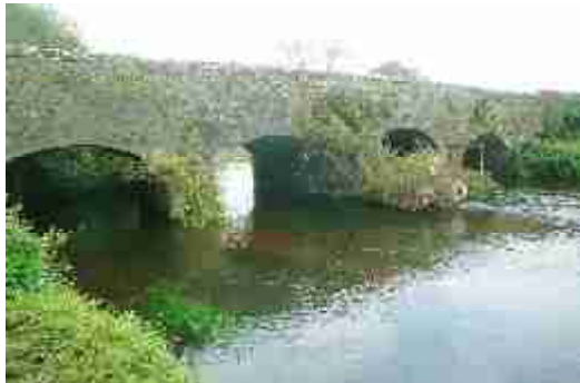
LAIAR-035-002_03 FWH 28/09/2007 Downstream (S) elevation from SW.
