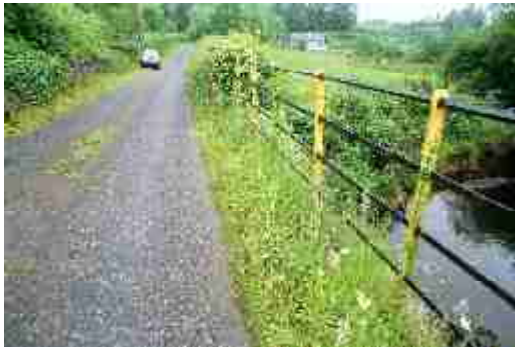
LAIAR-015-001_03 FWH 14/06/2007 Railing detail on downstream (E) side.
