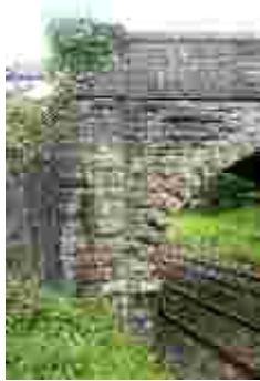
LAIAR-012-017_03 FWH 14/06/2007 Soffit detail. Note skew-laid bricks.
