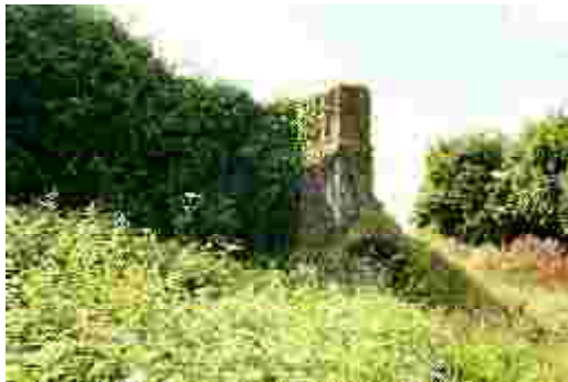
LAIAR-008-022_03 FWH 14/06/2006 Debicot Bridge: north-east terminal pier detail.
