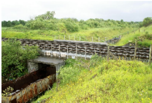
LAIAR-012-021_03 FWH 14/06/2007 Peat wagons passing through bridge.
