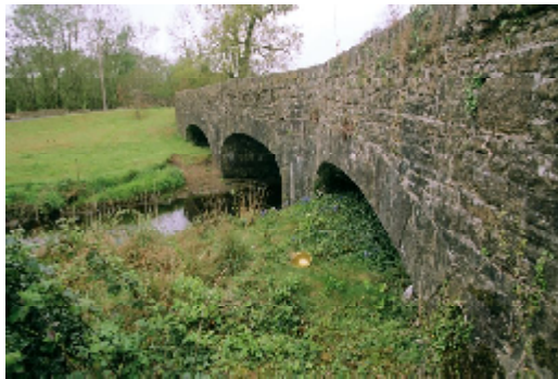
LAIAR-011-011_03 FWH 24/04/2007 Voussoir detail (downstream side of middle arch).
