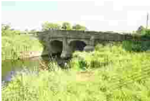
LAIAR-008-024_03 FWH 14/06/2006 Downstream (N) elevation.
