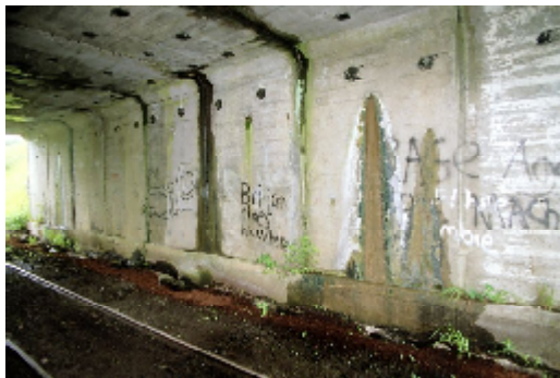
LAIAR-012-021_04 FWH 14/06/2007 Pre-cast concrete units.
