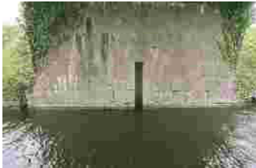
LAIAR-009-012_02 FWH 23/04/2007 Stop sluice slots in east side of abutment.
