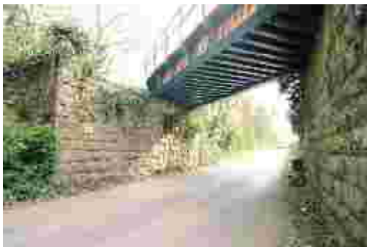
LAIAR-005-005_03 FWH 11/04/2007 Deck and east abutment detail, from NW.
