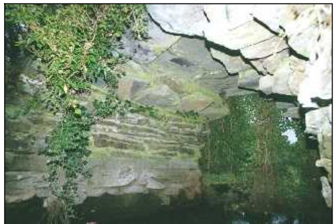
Fig 5.6 Corbelled span in Heywood Demesne (030-014).
