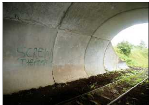
Fig 3.36b Road/rail bridge at Clonkeen showing early 2000s extension with pre-cast units (012-035).
