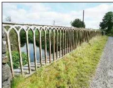
Fig 3.16 Railings on Derryduff Bridge.
