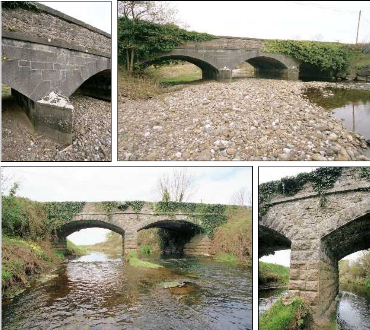
Fig 3.7a Top : Rathcoffey Bridge (003-011) on the Barrow, is a mid 1800s replacement of an earlier bridge (possibly the one on Moll's 1714 map (fig 3.1). It is virtually identical to Tinnahinch Bridge (003-014) just upstream. Fig 3.7b Bottom : Bay Bridge (004-001) also on the Barrow, has abutments of rock-faced blocks set in courses, as well as a string course and rusticated quoins and voussoirs.
