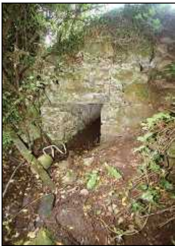
Fig 2.11 Derrygoony Bridge, a 60cm wide stone slab culvert at Garranmaconly (021-015).
