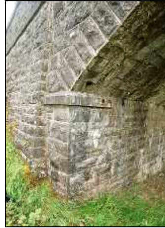
Fig 3.24 Road/rail bridge at Grange Beg (022-009). Note the high quality stonework even though it is on a very minor road.
