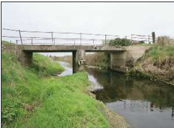
Fig 2.20a (left): Simple twin-span reinforced-concrete slab road bridge over Barrow at Cappaneary (003-043). Fig 2.20b (right): Strand Bridge is a reinforced-concrete beam and slab replacement of a previous bridge over a tributary of the Fushoge River at Ballickmoyler (032-006).
