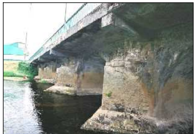
Fig 6.2 Cantilevered concrete footpath, Barrow Bridge (005-001).
