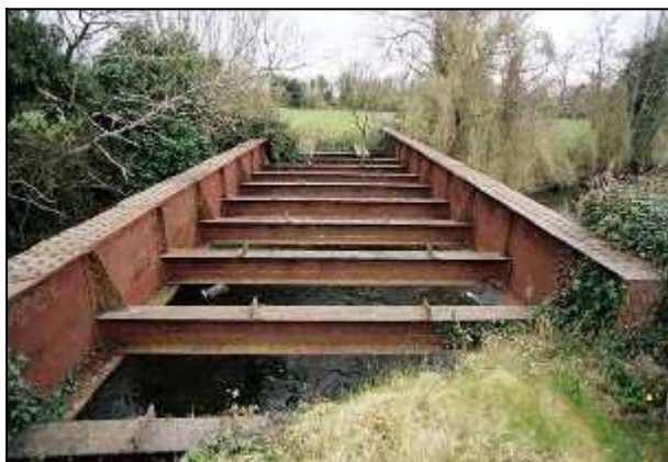
Fig 2.14a Left : The two principal girders of this rail/river bridge of 1885 on the Mountmellick Branch of the Great Southern & Western railway are of riveted steel plate (008-005). The track was carried on top of the smaller riveted I beams set between the girders' bottom flanges. Fig 2.14b Right : The main girders of Lacca Bridge over the Delour River are also of riveted metal plates (011-009). The bridge was fabricated c.1900 by an English firm and is the only one of its kind in the county.
