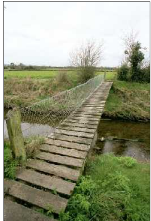
Fig 2.10 Modern timber footbridge at Cappaneary (003-044).
