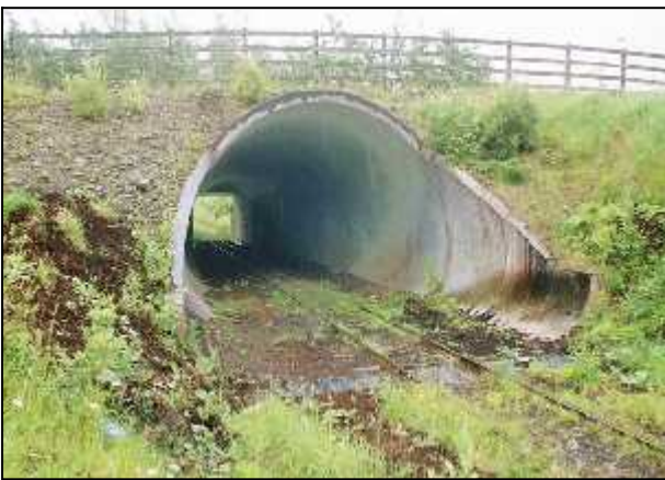
Fig 3.36b Road/rail bridge at Clonkeen showing early 2000s extension with pre-cast units (012-035).
