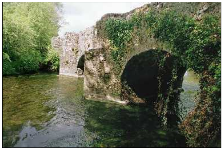
Fig 3.3 Ballykilcavan Bridge on the Stradbally River (014-038).
