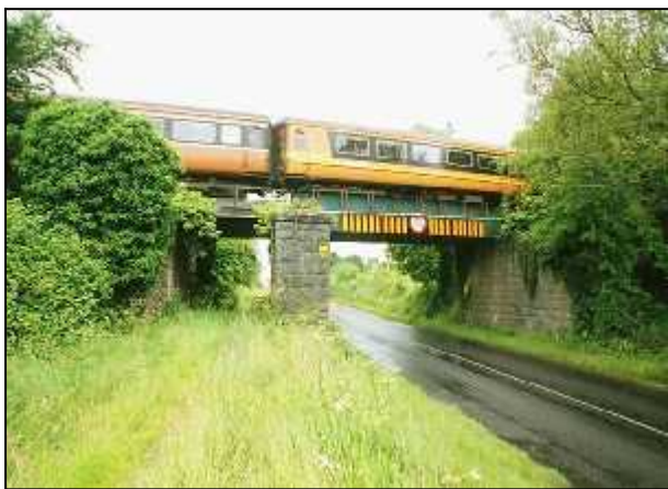
Fig 2.2 Examples of railway bridges. Top left: Rail/road bridge, Portlaoise (013-027). Top right: Rail/river bridge, Portlaoise (013-029). Bottom left: Rail/canal bridge, Cooltedery (005-006). The canal has been infilled hereabouts to create a road around Portarlinton.
