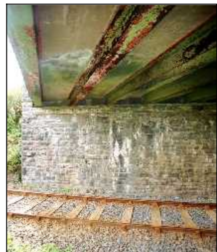
Fig 2.12a Left : Multiple RSJs support the concrete deck of Borness Bridge, a road/river bridge at Forest Lower (004-003). Fig 2.12b Right : Riveted I beams under deck of road/rail bridge at Shanboe (022-008).
