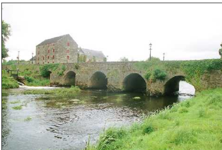
Fig 3.2 Upstream view of Castletown Bridge (016-015) showing the first phase of the present bridge. It was subsequently widened on its downstream side.
