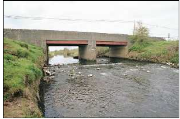
Fig 3.17a Left : Twin-span accommodation bridge at Cappanearry (003-043). Each of its slab spans measures c.4.56m (15ft). Fig 3.17b Right : Borneess Bridge, a twin-span public road bridge at Forest Lower (004-003). Because each span is 6.09m (20ft) and carries a heavier load than the accommodation bridge, the slab deck has metal beams underneath it.
