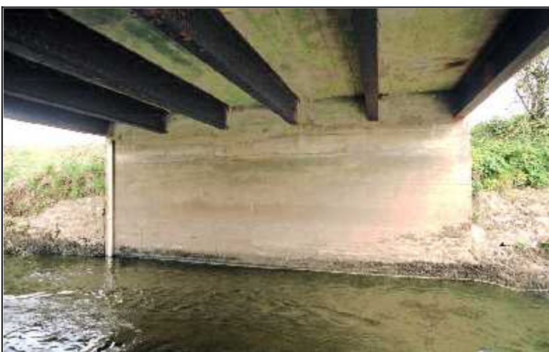
Fig 2.12a Left : Multiple RSJs support the concrete deck of Borness Bridge, a road/river bridge at Forest Lower (004-003). Fig 2.12b Right : Riveted I beams under deck of road/rail bridge at Shanboe (022-008).
