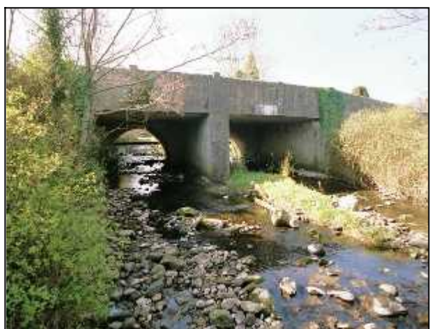
Fig 3.32 Left: Upstream view of Gorragh Bridge showing original stone bridge. Right: Downstream view showing 20 th century widening in concrete.
