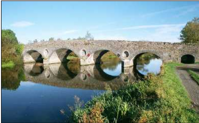
Fig 2.6 Maganey boasts the longest stone arch bridge in Laois. Five of its seven arches span the river; the remaining two are dry (026-020).
