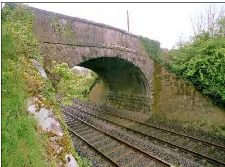
Fig 3.19a Top : Road/rail bridge at Ballymorris (005-024) with stepped voussoirs. Fig 3.19b Bottom : This nearby bridge at Tirhagar is similar but has radial voussoirs (005-030).
