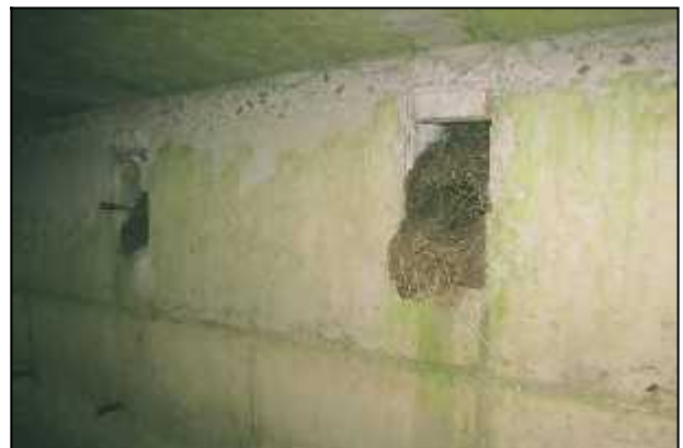
Fig 6.11 The falsework sockets under this concrete slab accommodation bridge at Paddock, near Mountrath, made ideal bird nesting sites (011-032).
