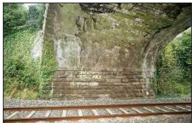
Fig 2.7a (left): GSWR road-over-rail bridge with skewly laid brick soffit at Kilbride (004-015). Fig 2.7b (right): A similar bridge at Corraun, but with a skew stone soffit (022-017).
