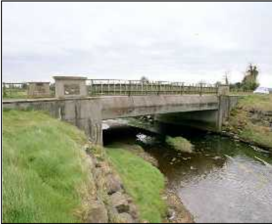
Fig 3.33 Ballyclare Bridge, a reinforced-concrete bridge comprising inverted T beams and slab deck (003-002). The plaque records its opening in February 1991 by Laois County Council.
