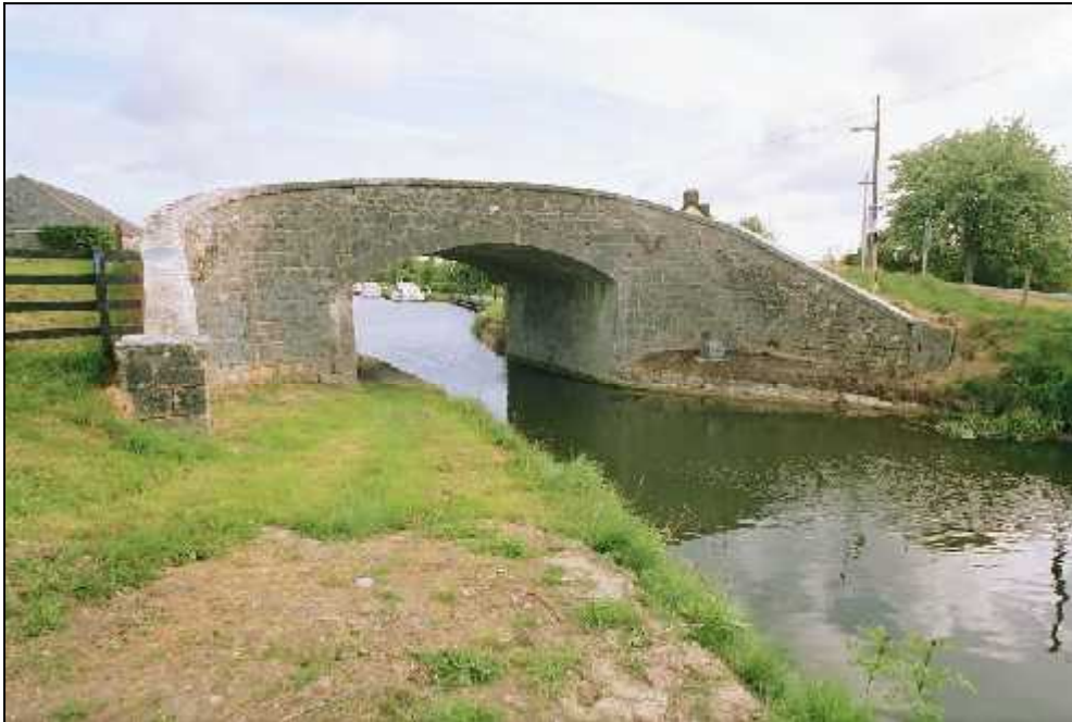
Fig 3.9 Vicarstown Bridge (014-008). Note the towpath through the arch on the left bank.
