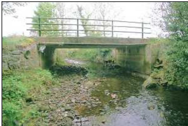
Fig 6.11 The falsework sockets under this concrete slab accommodation bridge at Paddock, near Mountrath, made ideal bird nesting sites (011-032).
