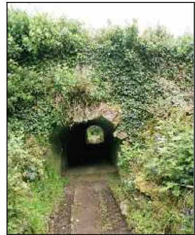
Fig 3.14 Pedestrian underpass at Ballykilcavan (014-018).
