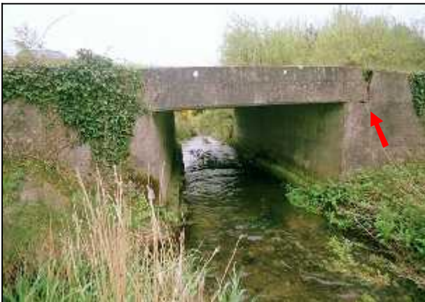
Fig 6.5a Above left : Collapsed parapet end on road bridge in Longford townland (016-038).
