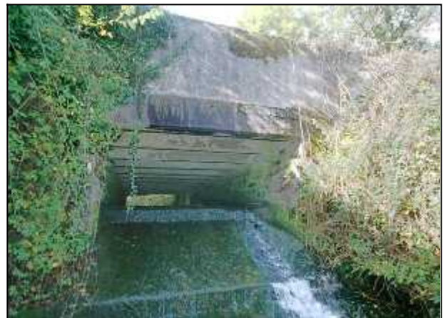
Fig 2.20a (left): Simple twin-span reinforced-concrete slab road bridge over Barrow at Cappaneary (003-043). Fig 2.20b (right): Strand Bridge is a reinforced-concrete beam and slab replacement of a previous bridge over a tributary of the Fushoge River at Ballickmoyler (032-006).
