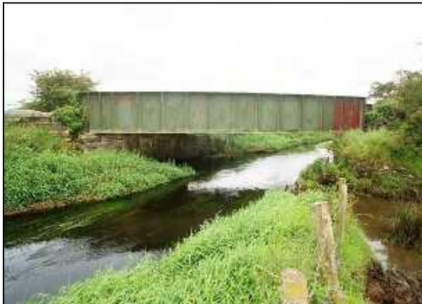
Fig 3.25 Railway bridge over the Nore at Curraghmore (021-005). Its skew deck spans 15.3m (50ft).
