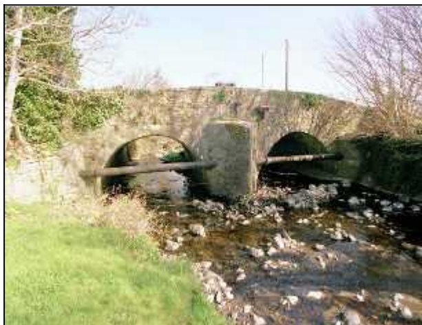
Fig 3.32 Left: Upstream view of Gorragh Bridge showing original stone bridge. Right: Downstream view showing 20 th century widening in concrete.
