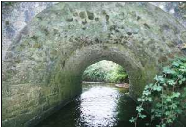
Fig 6.1a Left : The earlier narrow section of the original Attanagh Bridge is clearly visible through the arch of its widened section (035-009). Fig 6.1b Right : The slab concrete widened section of New Bridge is clearly evident against the masonry arches of the original bridge (021-008).
