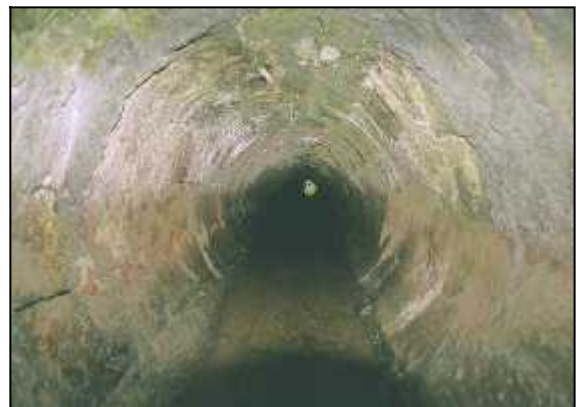
Fig 2.24 Stone pipe culvert 1.2m (4ft) dia under Athy Canal at Kullinure (009-017).
