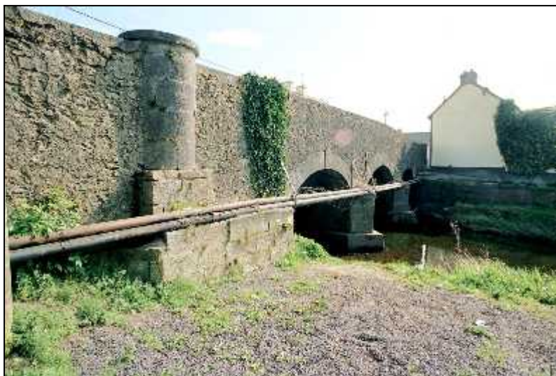
Fig 6.8 These water pipes detract from the appearance of Convent Bridge, Mountmellick (008-016).
