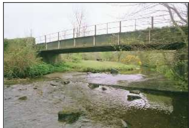
Fig 2.14a Left : The two principal girders of this rail/river bridge of 1885 on the Mountmellick Branch of the Great Southern & Western railway are of riveted steel plate (008-005). The track was carried on top of the smaller riveted I beams set between the girders' bottom flanges. Fig 2.14b Right : The main girders of Lacca Bridge over the Delour River are also of riveted metal plates (011-009). The bridge was fabricated c.1900 by an English firm and is the only one of its kind in the county.
