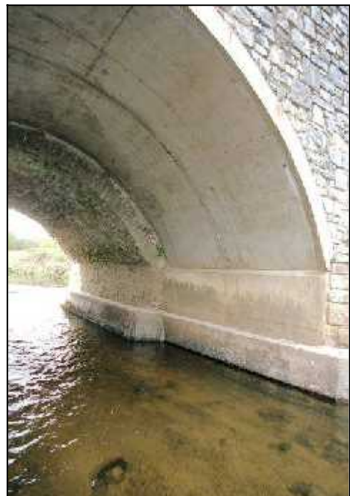
Fig 2.9a Top left : Downstream view of New Bridge (029-029) showing extension. Top right : Juxtaposition of stone and concrete arches on New Bridge. Fig 2.9b Bottom left : Downstream view of Spa Bridge (005-002). Bottom right : Concrete arch segments in Spa Bridge.
