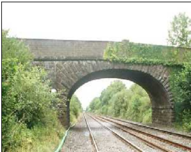
Fig 6.7 Left : The concrete block parapet to this road/rail bridge is in contrast to the high quality stonework of the original bridge (022-015). Right : Although this rebuilt parapet's stonework has been carefully laid, the weather-struck cement-rich pointing detracts from its appearance (003-028).
