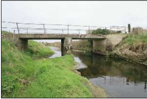
Fig 3.17a Left : Twin-span accommodation bridge at Cappanearry (003-043). Each of its slab spans measures c.4.56m (15ft). Fig 3.17b Right : Borneess Bridge, a twin-span public road bridge at Forest Lower (004-003). Because each span is 6.09m (20ft) and carries a heavier load than the accommodation bridge, the slab deck has metal beams underneath it.
