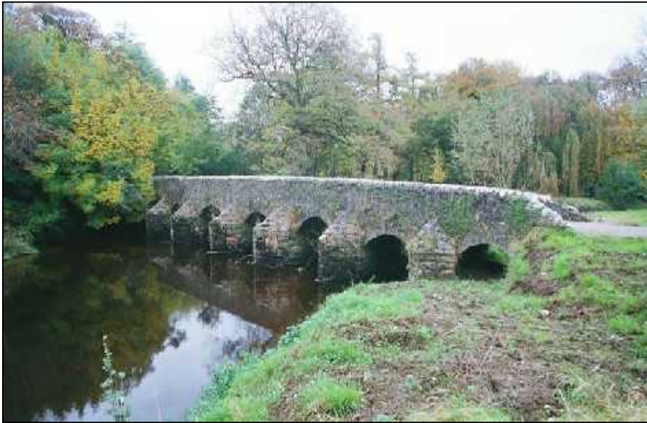
Fig 2.4 The eight-arched Knapton Bridge in Abbeyleix Demesne (029-004).
