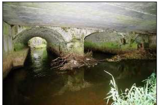
Fig 6.1a Left : The earlier narrow section of the original Attanagh Bridge is clearly visible through the arch of its widened section (035-009). Fig 6.1b Right : The slab concrete widened section of New Bridge is clearly evident against the masonry arches of the original bridge (021-008).
