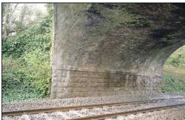
Fig 2.7a (left): GSWR road-over-rail bridge with skewly laid brick soffit at Kilbride (004-015). Fig 2.7b (right): A similar bridge at Corraun, but with a skew stone soffit (022-017).
