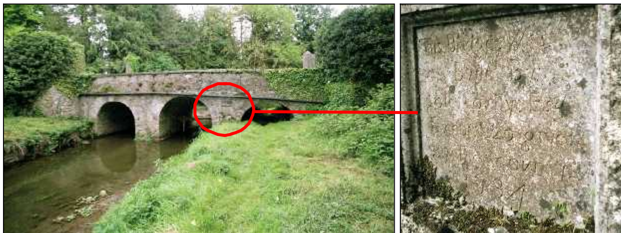
Fig 3.5 Pole's Bridge, Stradbally, with plaque commemorating its builder Pole Cosby (019-011).
