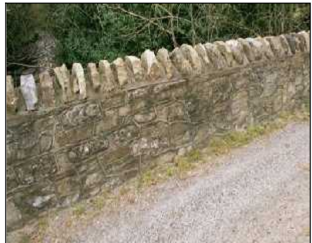
Fig 6.7 Left : The concrete block parapet to this road/rail bridge is in contrast to the high quality stonework of the original bridge (022-015). Right : Although this rebuilt parapet's stonework has been carefully laid, the weather-struck cement-rich pointing detracts from its appearance (003-028).
