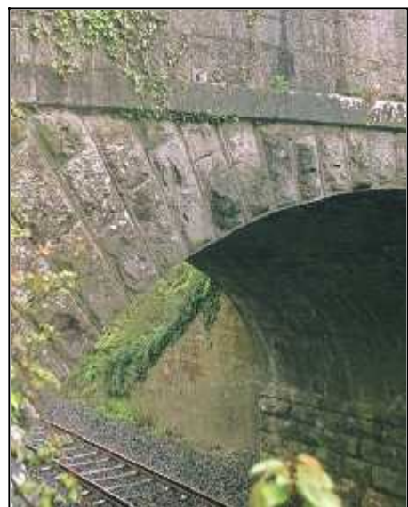
Fig 3.19a Top : Road/rail bridge at Ballymorris (005-024) with stepped voussoirs. Fig 3.19b Bottom : This nearby bridge at Tirhagar is similar but has radial voussoirs (005-030).
