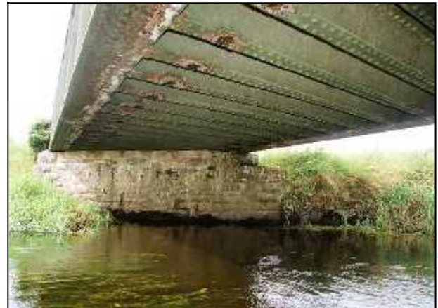
Fig 3.25 Railway bridge over the Nore at Curraghmore (021-005). Its skew deck spans 15.3m (50ft).
