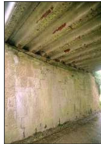
Fig 2.17 Riveted longitudinal metal troughing at a rail/road bridge at Clonanny (005-037).
