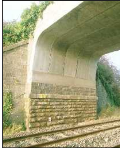
Fig 2.21a ( left ): Standard pre-cast beams on new road bridge over Cork line at Cuddagh (022-020). This bridge replaced the original level-crossing.
