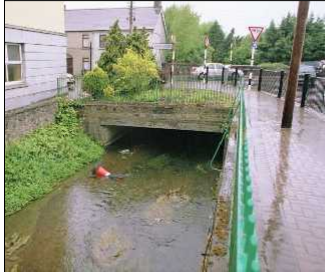
Fig 3.29 Concrete slab road bridge over Triogue River at the east end of Portlaoise (013-069).
