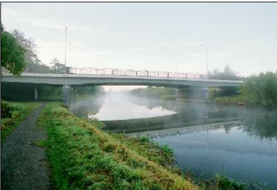
Fig 2.22 The Bill Duggan Bridge, opened in 1999 on the northern outskirts of Carlow town (032-032).
