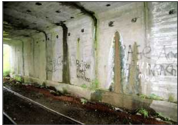
Fig 3.36c Rail/rail bridge at Clonkeen showing pre-cast concrete units (012-021).
