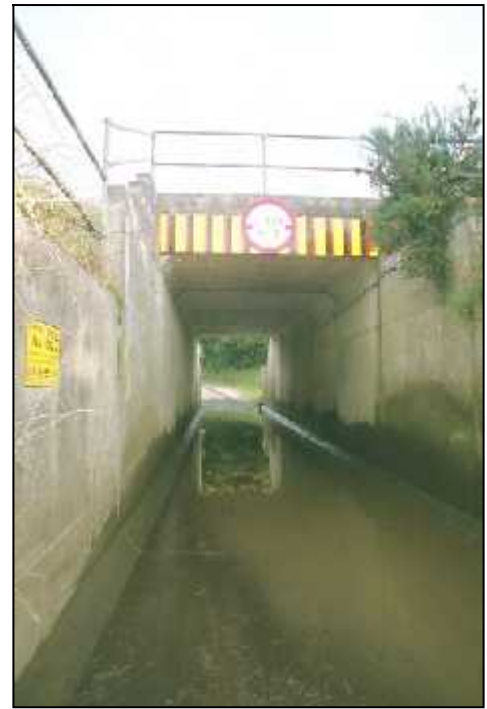
Fig 3.37 Underbridge at Rathnaleugh on the Dublin-Cork railway line (027-007).
