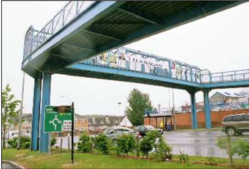
Fig 2.19 Footbridge over bypass, Portlaoise (013-068).
