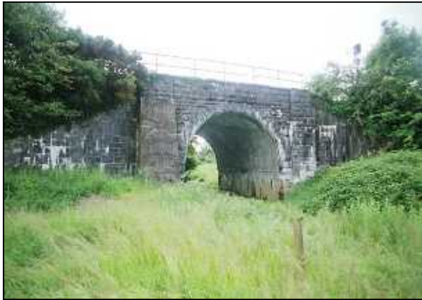
Fig 3.20a (left) Rail bridge over a tributary of the Nore at Clonadacasey (017-016). It spans 6.03m (20ft). Fig 3.20b (right): Rail bridge over Nore at Ballycleary; (017-030). The deck was originally of timber; each span exceeds 9m (30ft).
