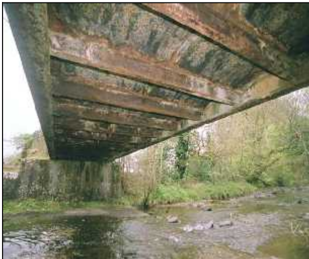
Fig 3.30a (left): Underside of Lacca Bridge showing transverse jack arches (011-009). Fig 3.30b (right): Underside of Birchgrove Bridge showing longitudinal jack arches (015-001).
