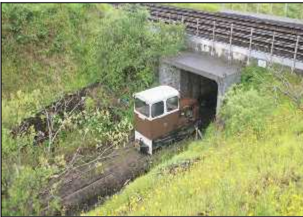
Fig 3.36c Rail/rail bridge at Clonkeen showing pre-cast concrete units (012-021).
