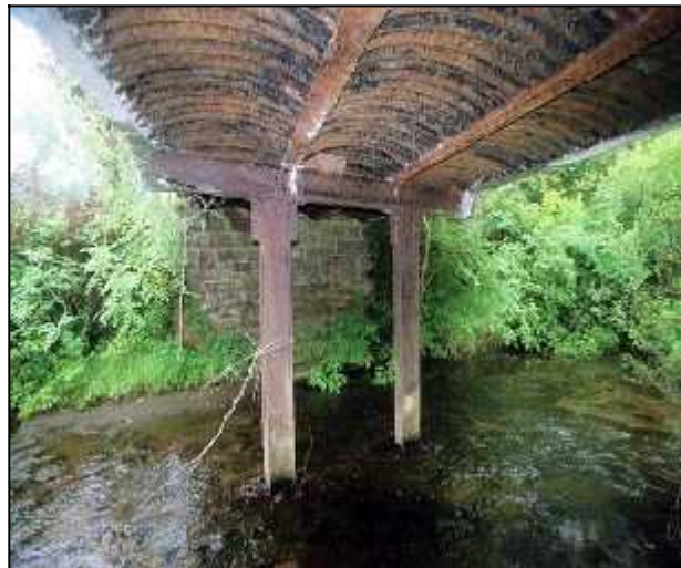
Fig 3.30a (left): Underside of Lacca Bridge showing transverse jack arches (011-009). Fig 3.30b (right): Underside of Birchgrove Bridge showing longitudinal jack arches (015-001).
