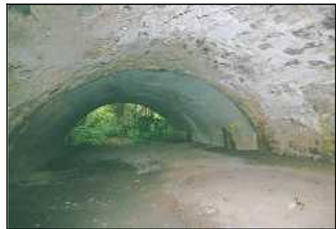
Fig 2.8 Crettyard Bridge over the Dinin is the best example in the county of a wholly-concrete arch bridge (31-029).
