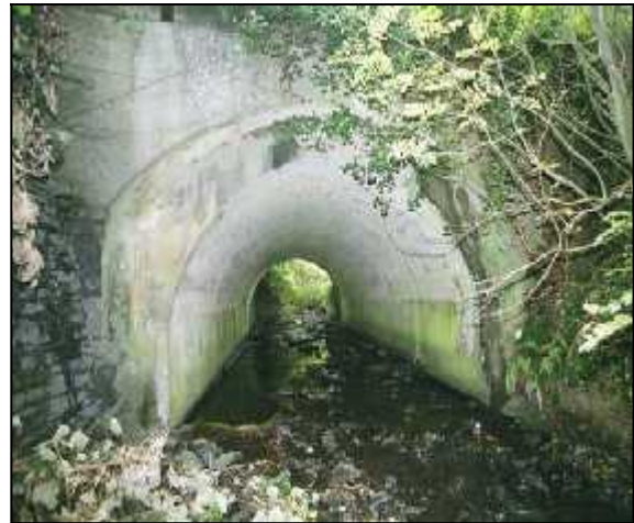
Fig 2.8 Crettyard Bridge over the Dinin is the best example in the county of a wholly-concrete arch bridge (31-029).
