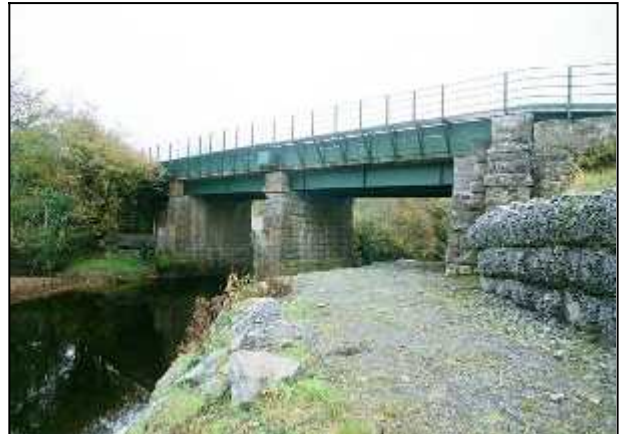
Fig 3.20a (left) Rail bridge over a tributary of the Nore at Clonadacasey (017-016). It spans 6.03m (20ft). Fig 3.20b (right): Rail bridge over Nore at Ballycleary; (017-030). The deck was originally of timber; each span exceeds 9m (30ft).
