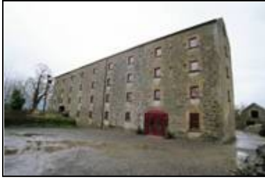
LAIAR-029-020_05 16/02/2006 East façade, from south-east.
