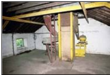
LAIAR-019-001_13 11/08/2005 No.1 kiln firehole.
