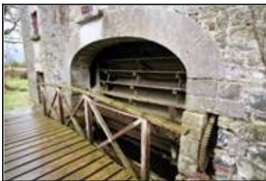
LAIAR-029-020_08 16/02/2006 North end of east façade showing waterwheel and tailrace.
