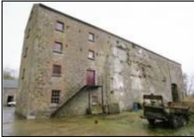
LAIAR-029-020_06 16/02/2006 Remains of east wall of kiln block (looking at inside face).
