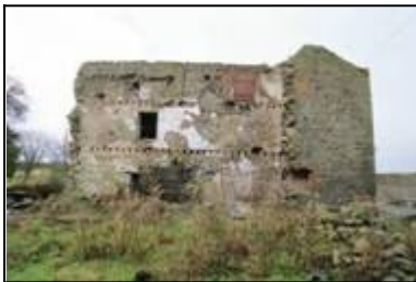
LAIAR-029-020_07 16/02/2006 Waterwheel sluice gate.
