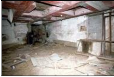
LAIAR-016-014_07 26/08/2005 Second floor of corn mill, looking north.
