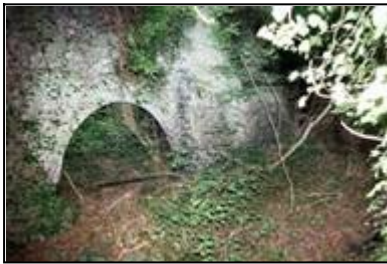
LAIAR-014-017_01 12/08/2005 Internal view looking south-east from north-west corner.
