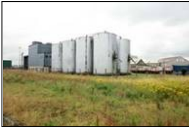
LAIAR-005-010_08 28/07/2005 View of site from north-east.
