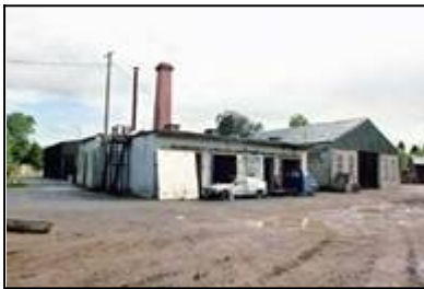
LAIA R-029-006_06 24/08/2005 Roof of drying kilns, with chimneys behind. Note ventilators.
