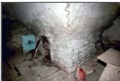
LAIAR-028-004_10 25/08/2005 Ground floor of kiln at south end of malt house.
