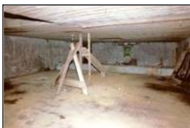
LAIAR-008-032_07 29/07/2005 Bottom end of elevator at north end of malt house.
