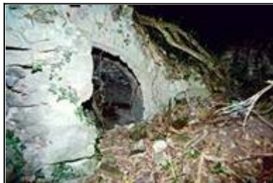
LAIAR-014-017_02 12/08/2005 Remains of kiln vaulting at south end of mill.
