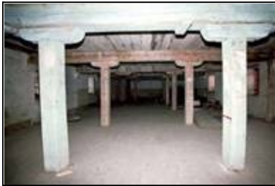
LAIAR-016-014_08 26/08/2005 Top two floors of corn mill, looking south.
