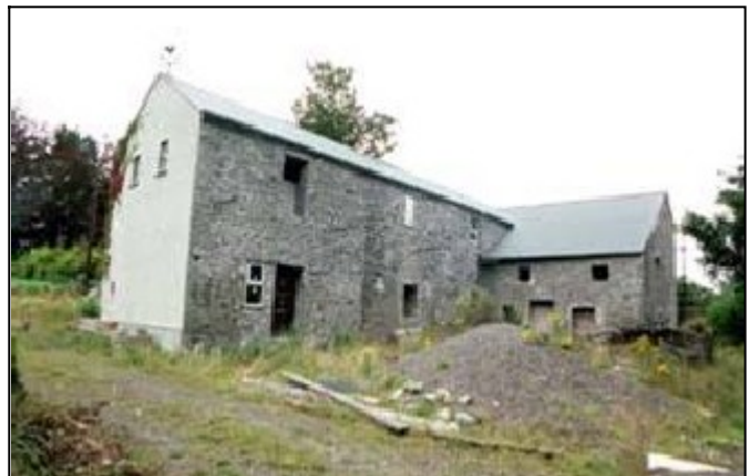
Fig 2.10 Knocknagroagh Mill (008-051) is typical of many traditional corn mills in Co Laois. The actual mill is at right, and the kiln and store at left.
