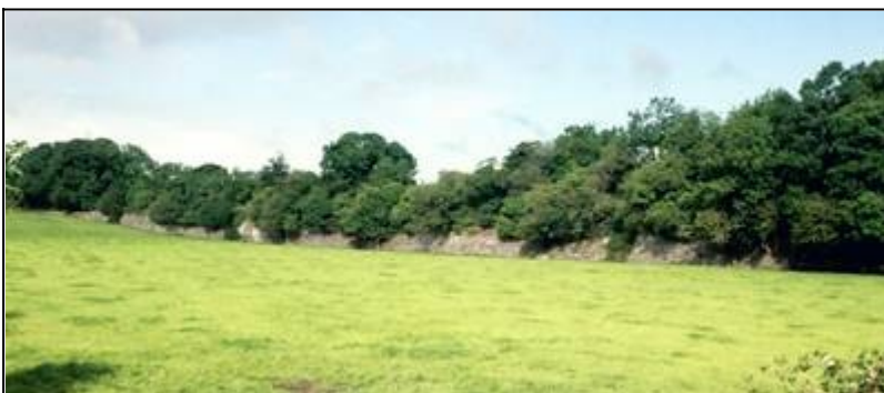
Fig 2.5 What appears to be an estate wall is in fact a 200m long revetted embankment of the headrace feeding Carrigh Mill, Kilnaseer (028-017). The resultant head of water was some 6m high by the time it reached the mill.
