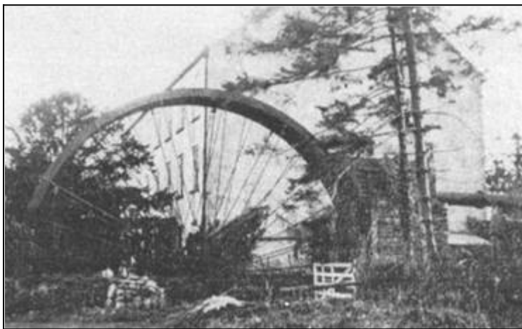
Fig 4.3 This photograph of Monordree Mill shows a spoked high breastshot waterwheel. There would have been a spur gear around its rim, with a bull-nut take-off to a shaft into the machinery ( O'Keefe, p.22 ).
