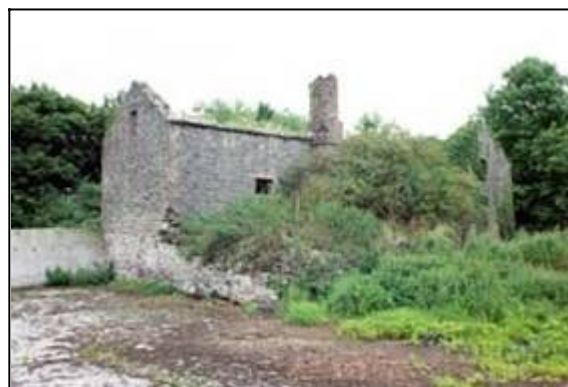
Fig 2.17 Remains of Simmons' steam mill, Ballylehane.
