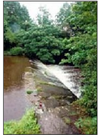
Fig 4.4 Weir on Owenass River.
