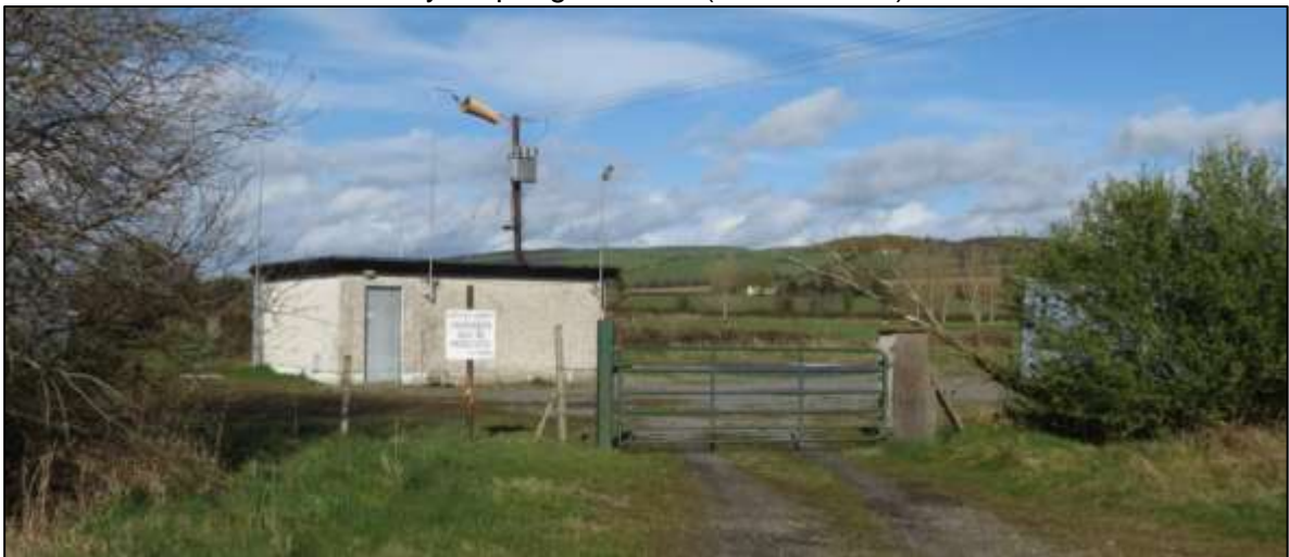
Entrance gate to Kyle Spring pump house and works, looking east.
