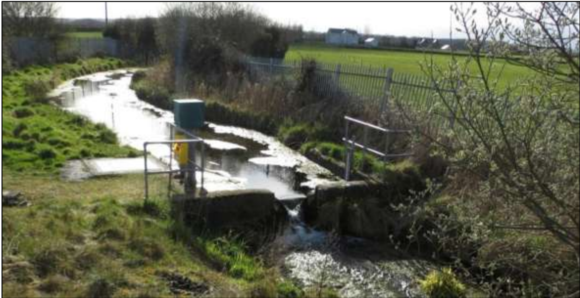
View of the spring and overflow, looking west towards Timahoe-Stradbally road.
