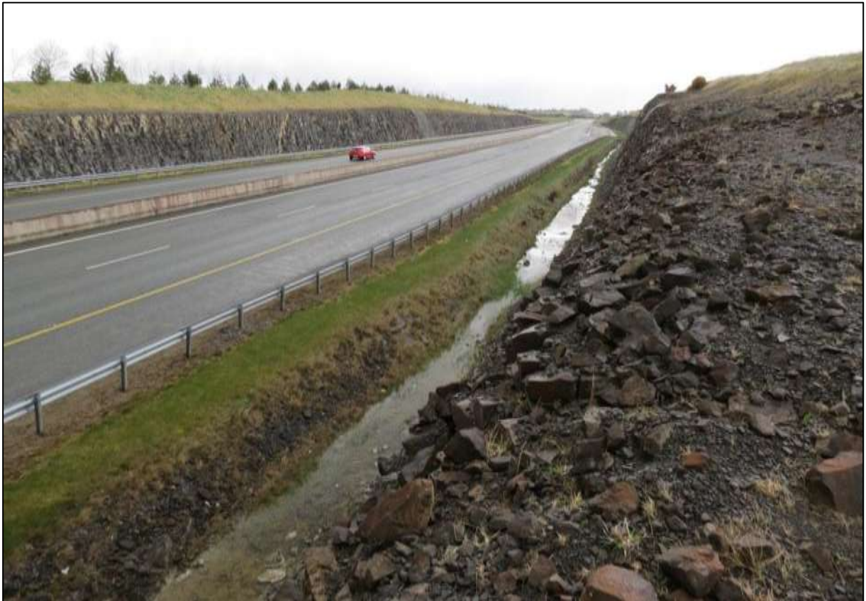
M7 Road Cut viewed looking east from top of southern embankment.
