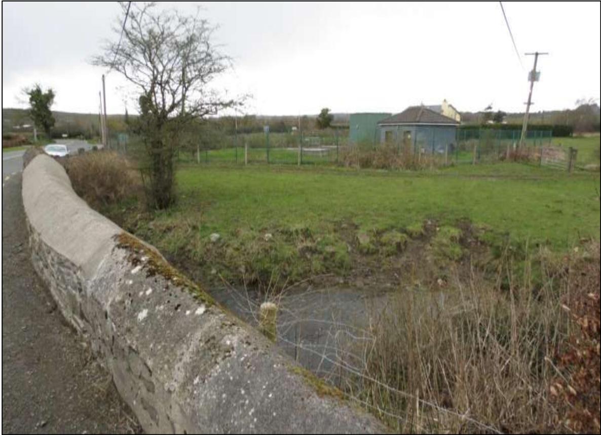
Swan Public Water Supply Scheme viewed from Swan Bridge.
