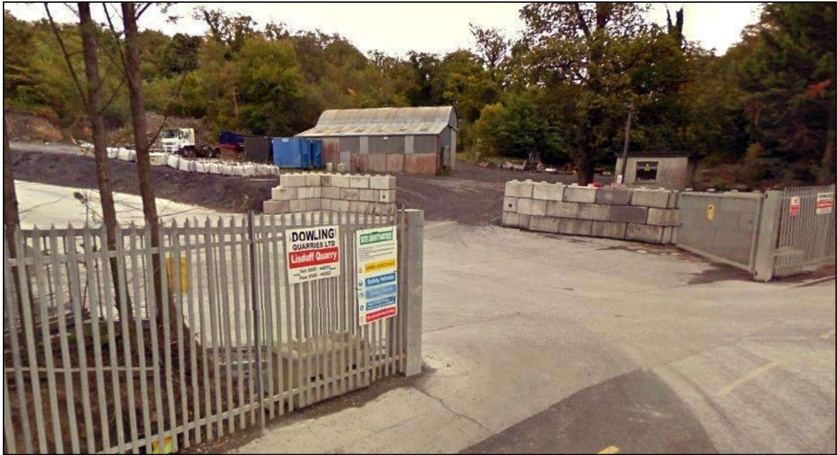
Entrance to Lisduff Quarry.
