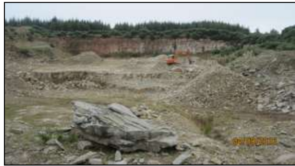
Inside Glebe Quarry.
