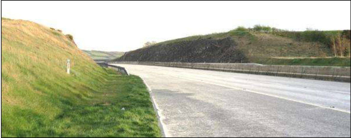
M8 Road cut viewed looking south from lay-by.
