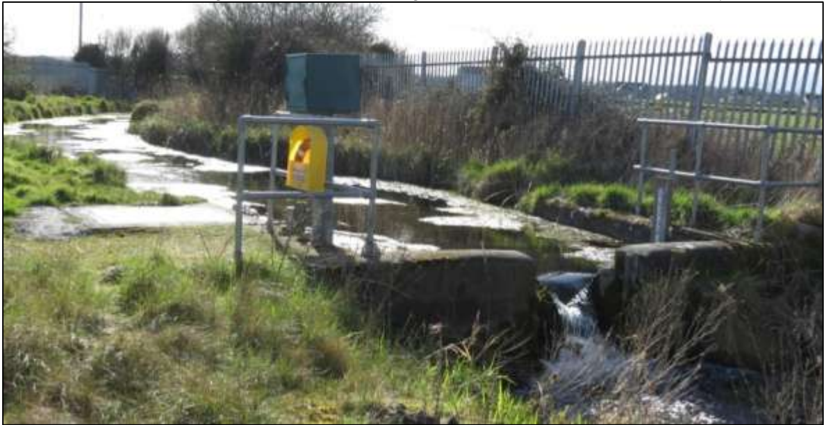
Kyle Spring overflow (all fenced off).
