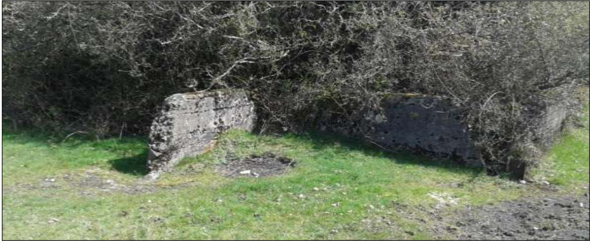
Remains of washing/screening plant at Modubeagh Mine.
