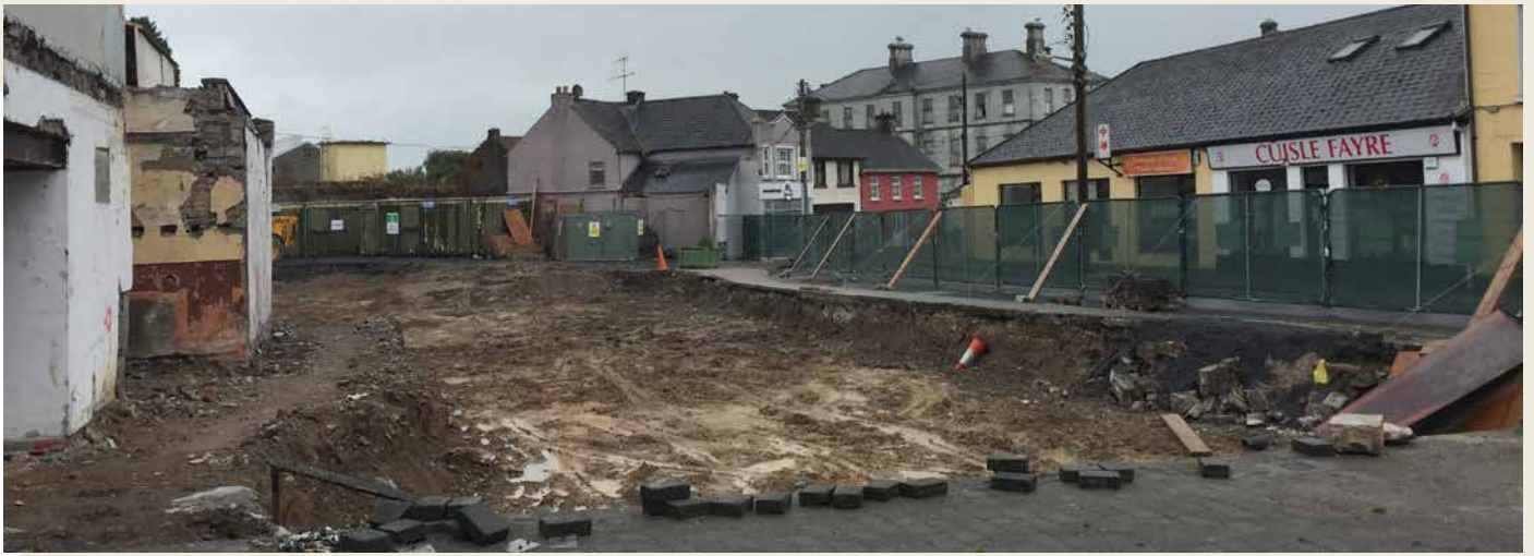
Fig. 99: Corner seen from lower square
