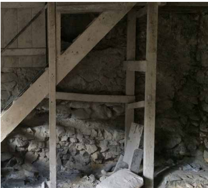
Fig. 55: Interior of fort wall within eastern structure
