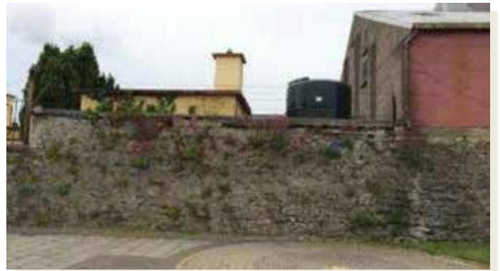
Fig. 42: Higher section of E wall adjoining mill site
