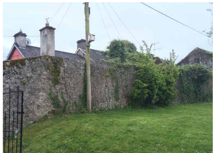
Fig. 108: Rears of Sites 21 and 21 seen from inside Fort
