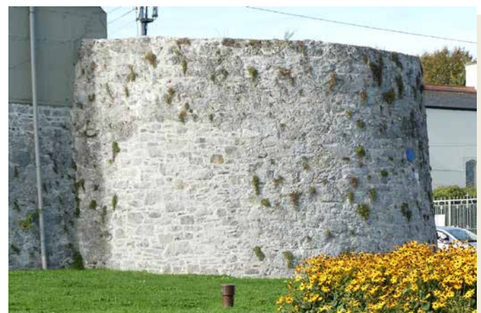
Fig. 48: Flanker or bastion with repaired breach
