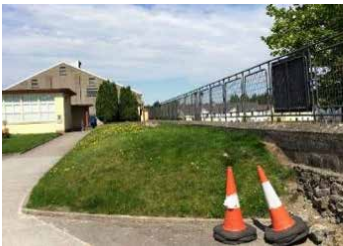
Fig. 43: Inner face of East wall with bank
