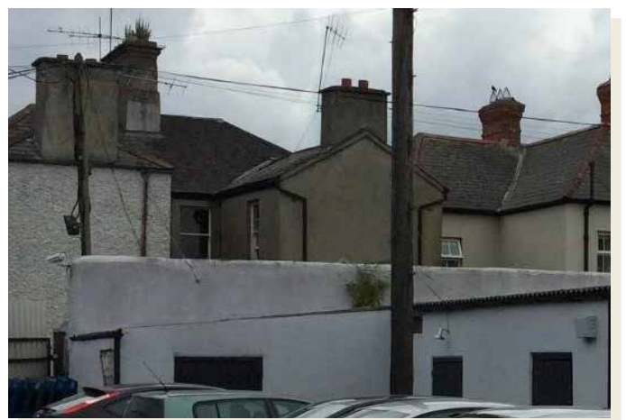
Fig. 74: Rear seen from interior of Fort
