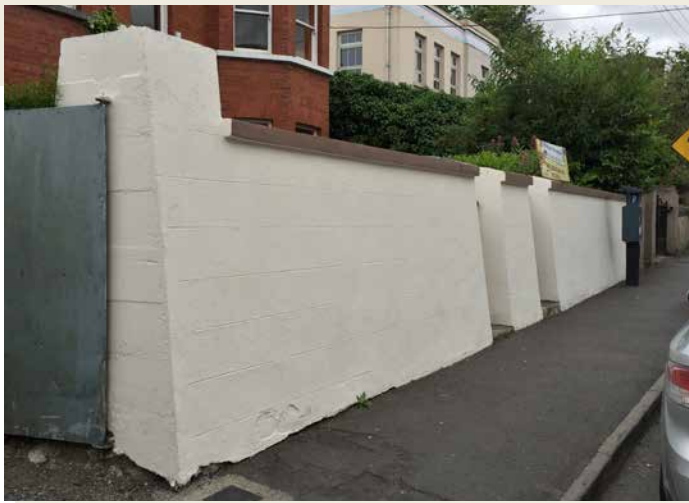
Fig. 59: Fort wall reconfigured as garden wall
