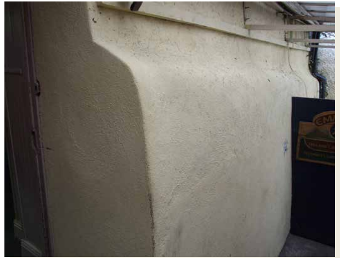
Fig. 90: Section of wall to rear of No. 29 within lobby to No. 30
