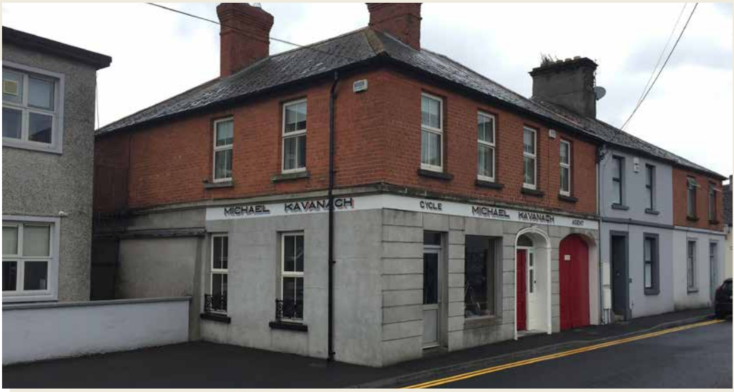
Fig. 69: View from Railway Street
