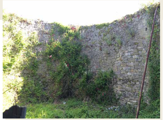
Fig. 49: Interior of round bastion
