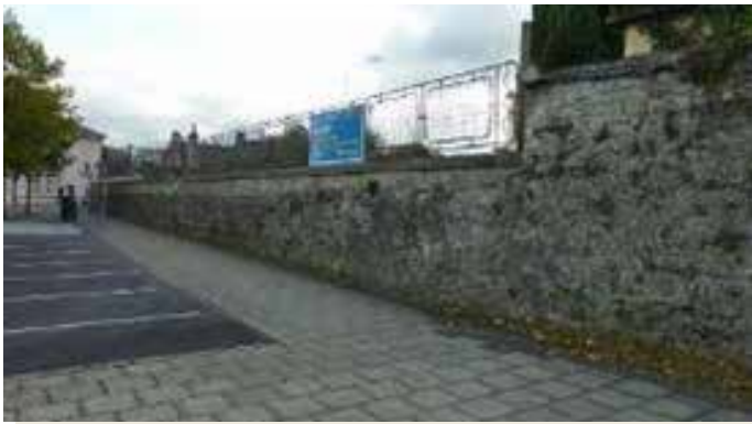
Fig. 41: External face of E wall, S end
