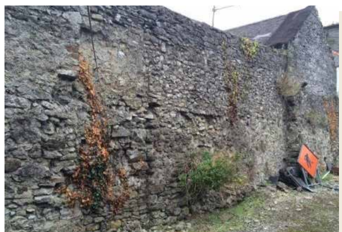
Fig.88: Detail of internal façade of west side of fort wall to the right of plate with later ope to left of plate
