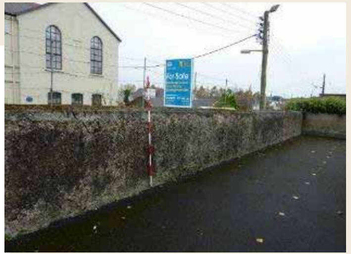
Fig. 40: Inner face of N wall
