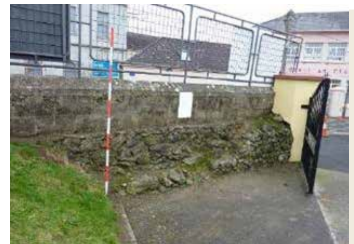
Fig. 44: Exposed section of E wall at school gateway
