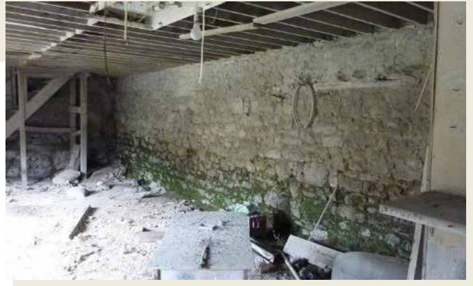
Fig. 54: Interior of eastern structure with eastern wall of early nineteenth-century date
