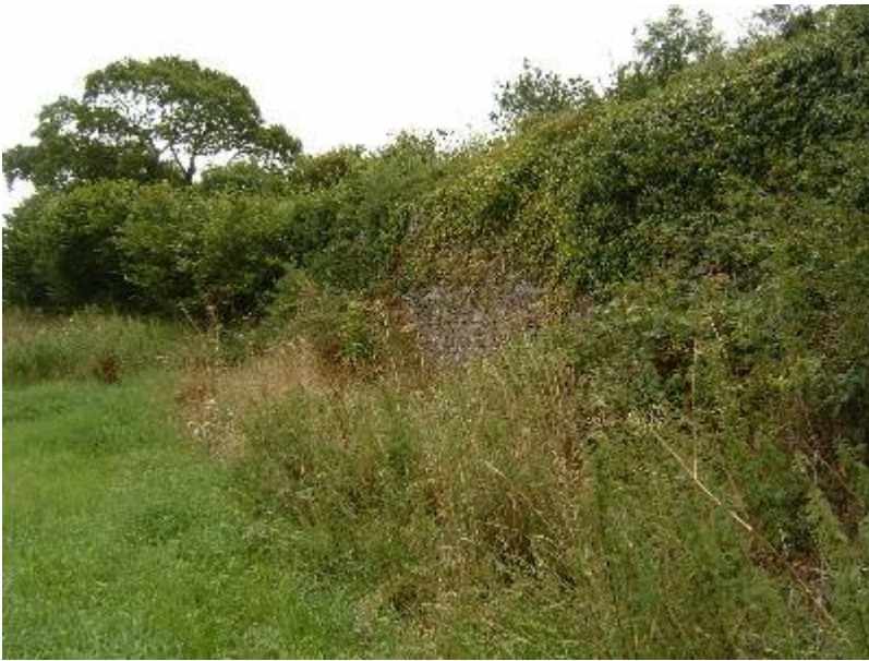
Plate 3.11 Old stone retaining wall along the Ridge Road
