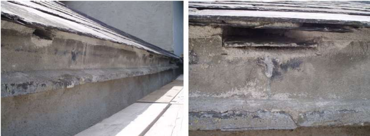
Figure 6.1: Artificial roost access slits under eaves suitable for Pipistrelle species and Whiskered bats (Bishop's Palace, Kilkenny)
