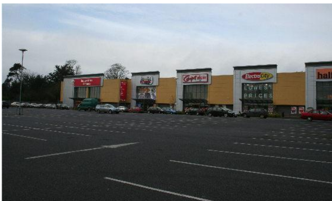
Fig. 5.9 Carlow Retail Park, Hanover, Carlow
