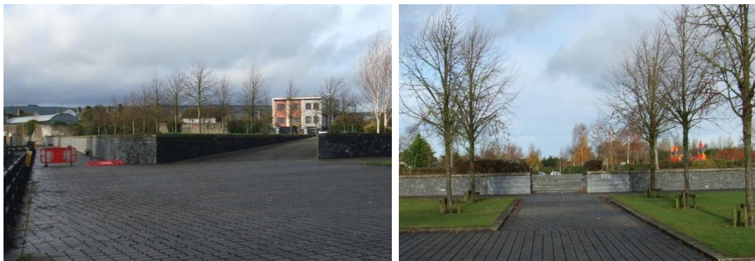
Figure 2-3 Flood Defences built into the landscaping of the Town Park
