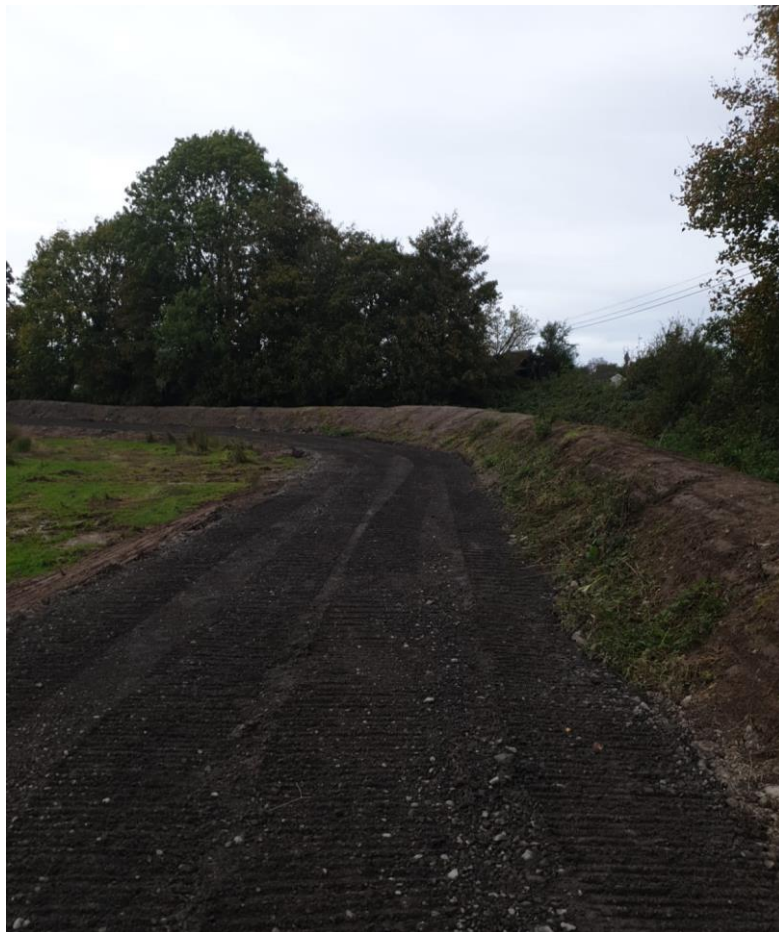
Drinagh Mill Race embankment repair
