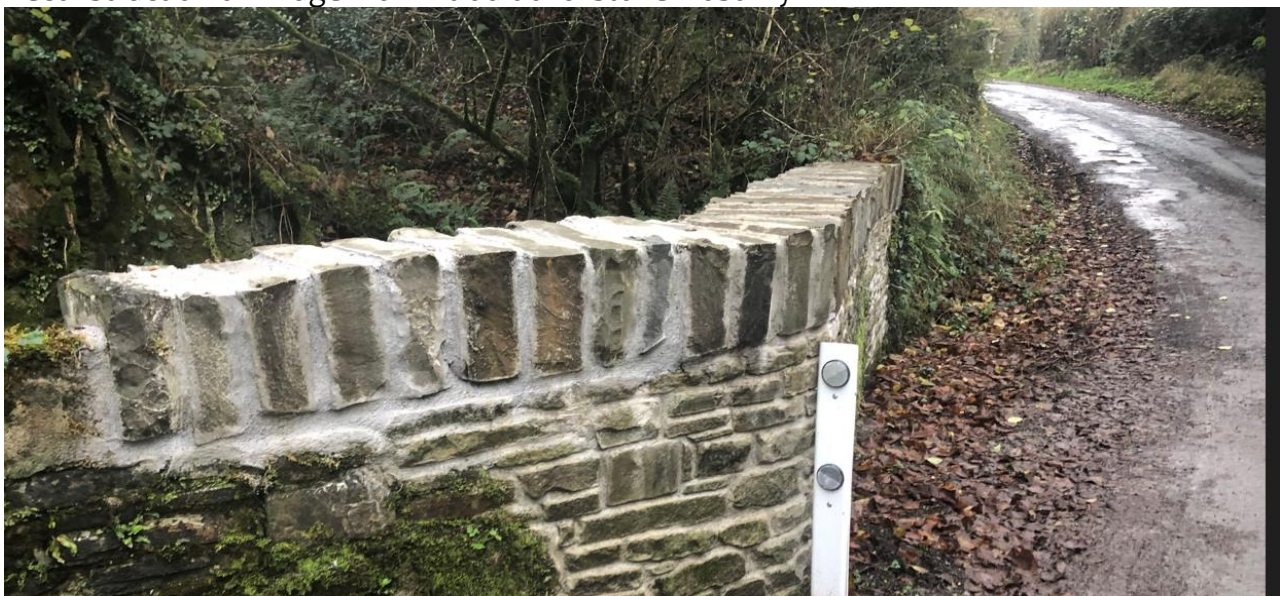
Reconstruction of Bridge Wall in traditional stone masonry
