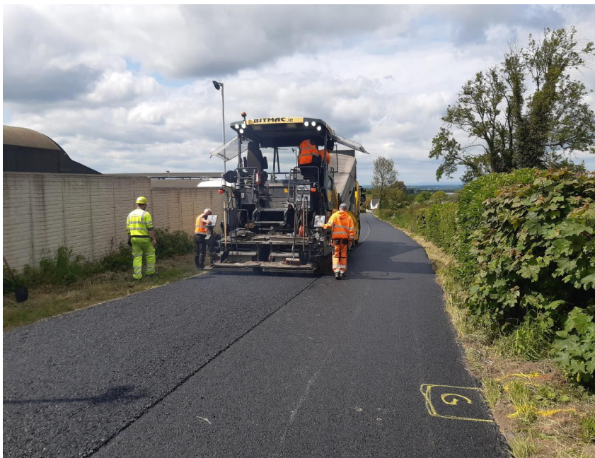
Restoration Improvement Works (Strengthening) on the L-27781 at Cloncullane Ballyroan
