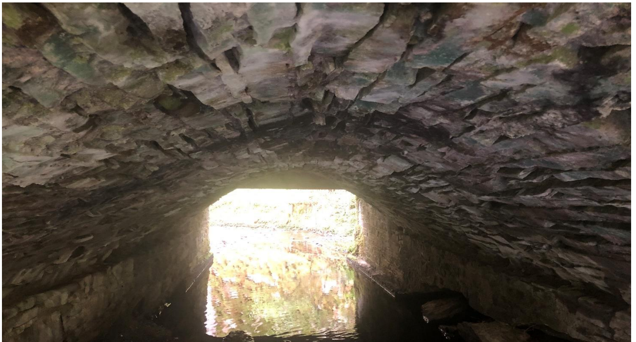
Before and after: Re-pointing of Arch soffit/barrell under Kilfeacle Bridge
