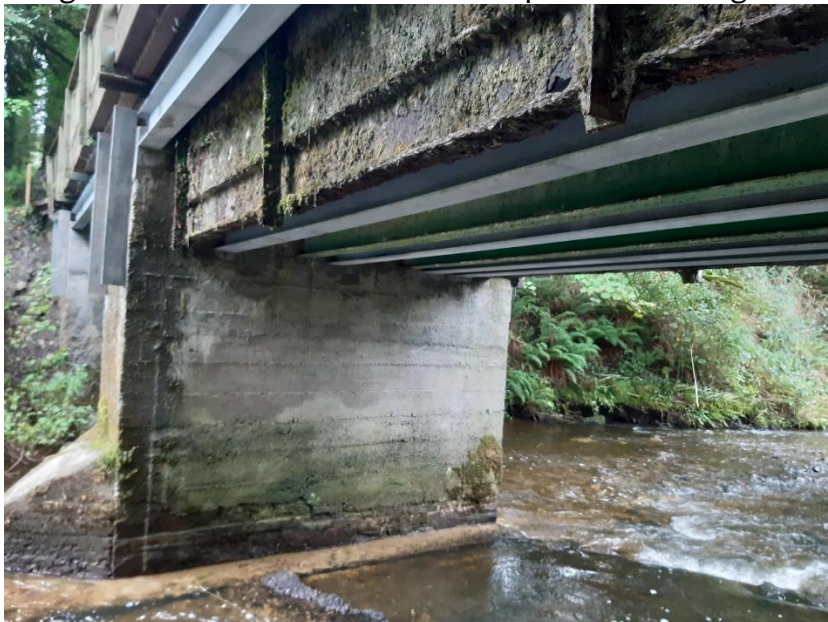
Additional reinforcement beams installed at Clohogue bridges Ballinakill
