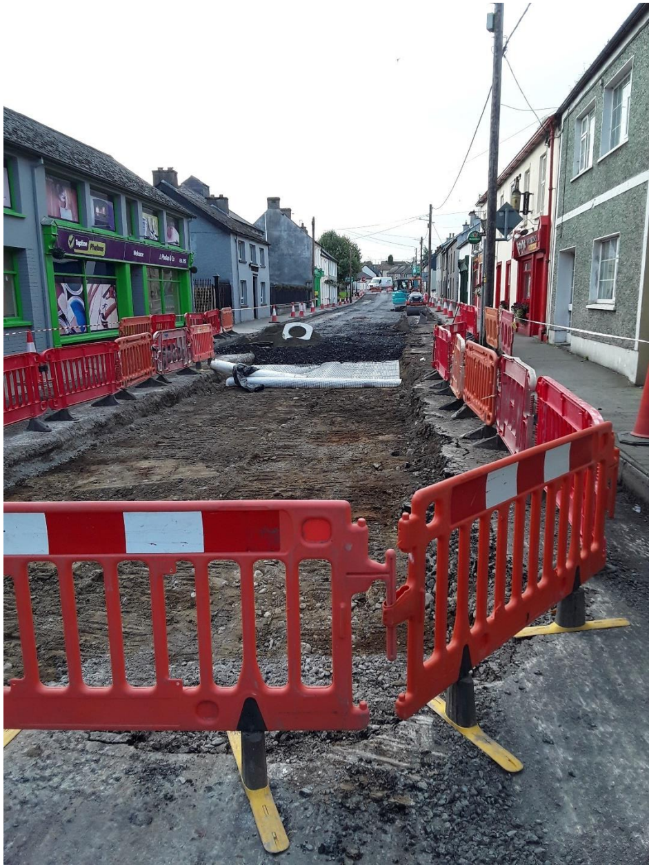
Pavement reconstruction Chapel Street, Durrow
