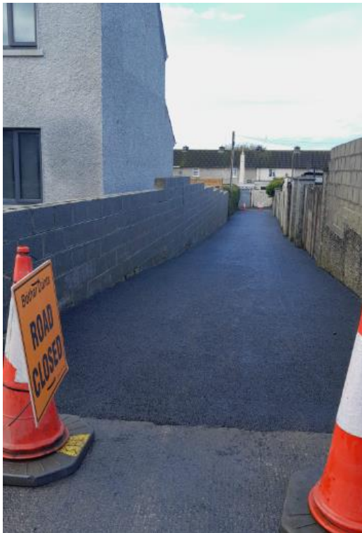
Road surfacing St. Brigid's Place Portlaoise
