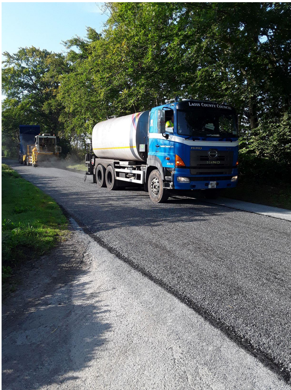
Surface Dressing at Portnahinch, Mountmellick
