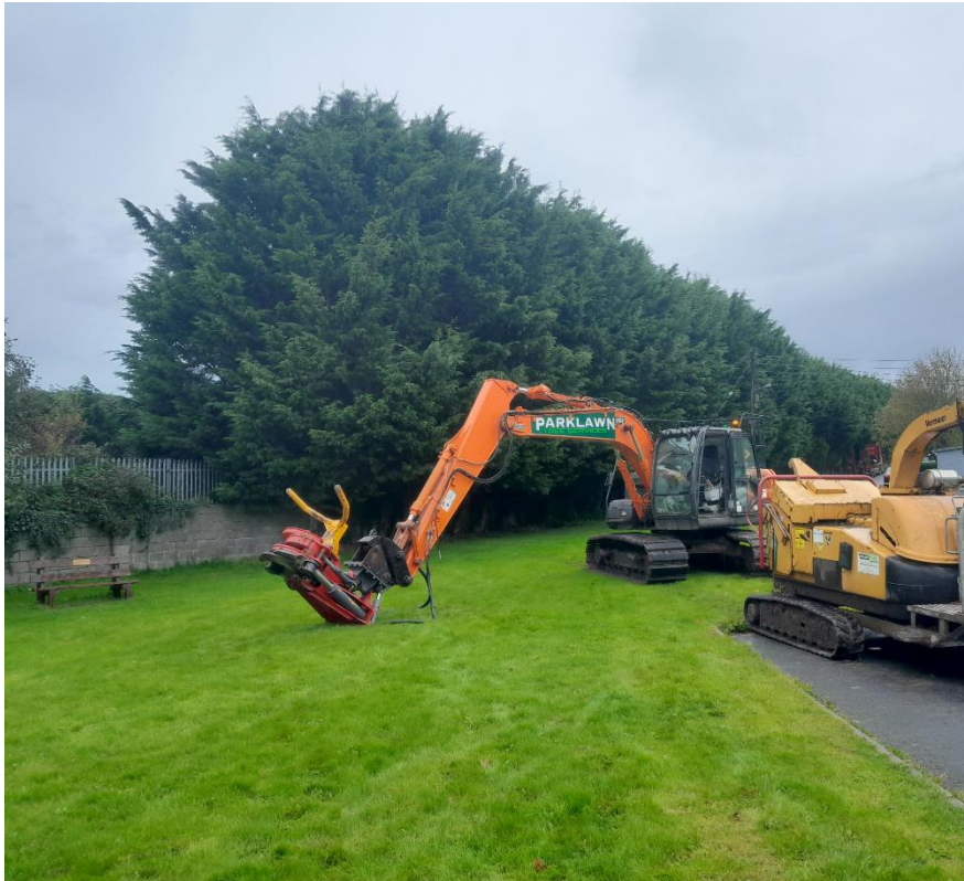
Tree management works in St Brigid's Place Portlaoise
