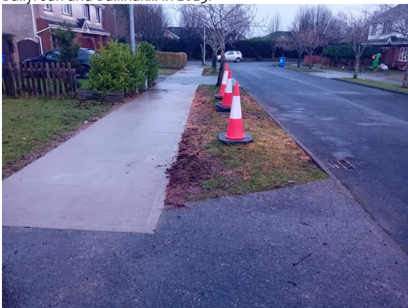
Footpath Replacement works in Woodgrove Portlaoise
