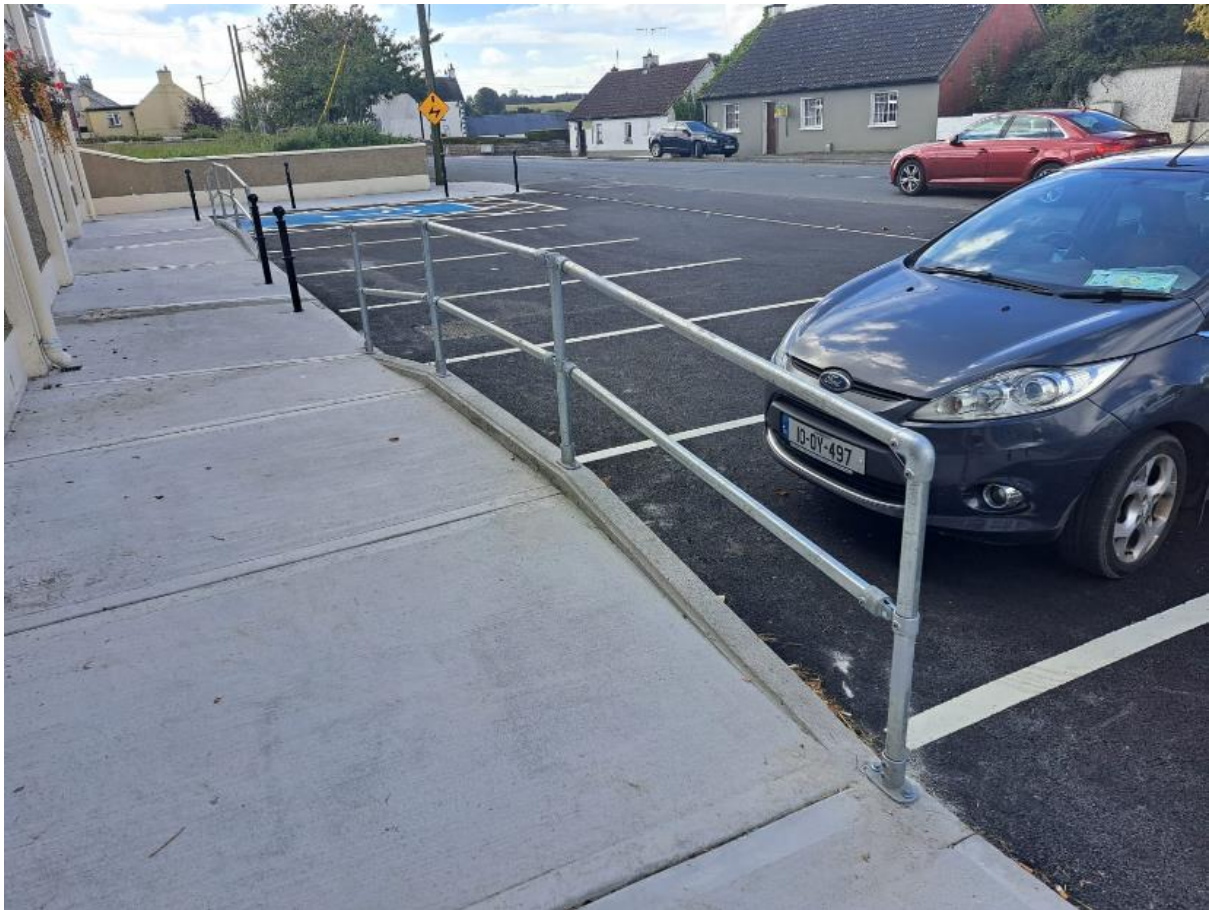
Drainage, resurfacing, and footpath works Main Street Ballyroan
