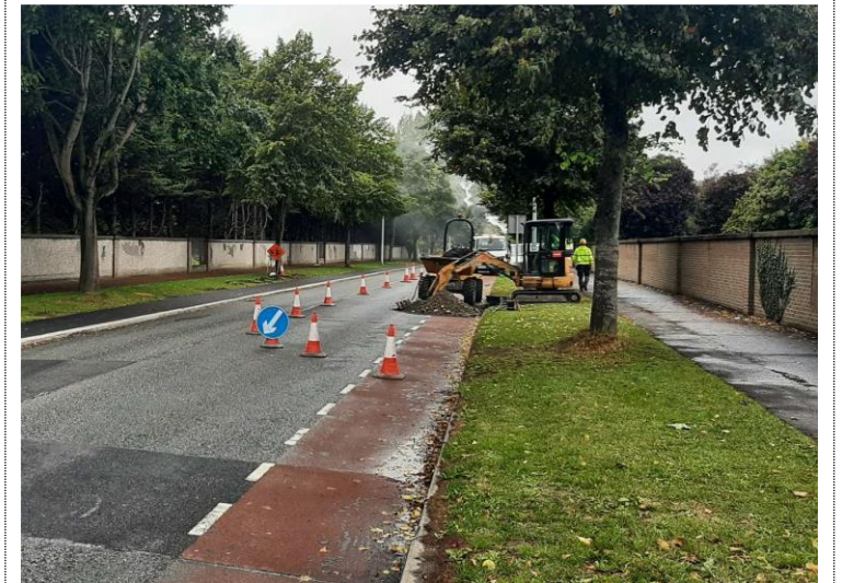
Step 1 Gully excavation
