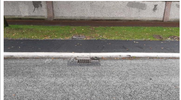
Step 3 New extruded kerb, asphalt cycleway and gully mastic surround
