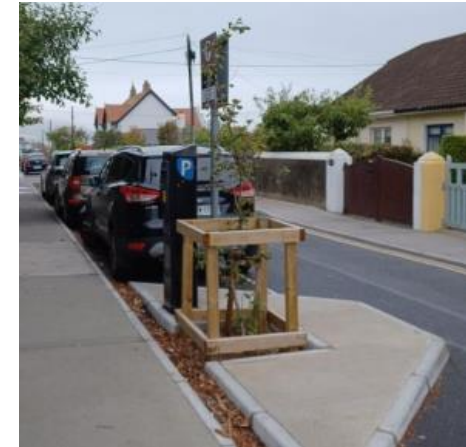
Tree Pit with drainage channel (Photo credit Wicklow CC)
