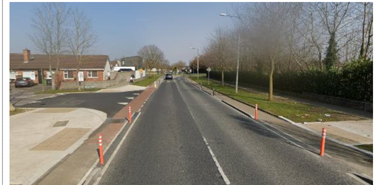
Phase 2 Concrete Build Out and Ramps ©Google Street View Mar 2022
