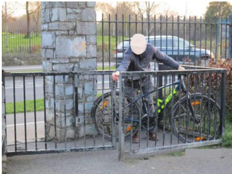
Figure 2: “Kissing Gates” are a restrictive form of Access Control
