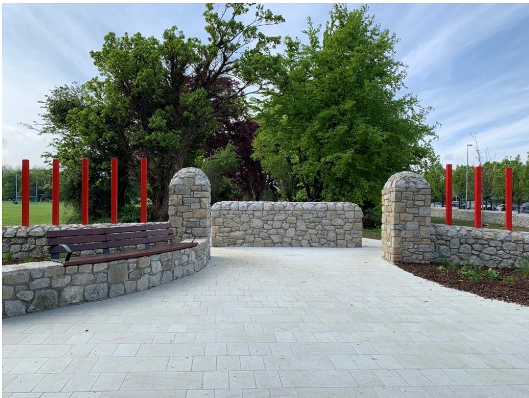
Figure 13: Example of welcoming access to an active travel route with a gap of 1.8m provided to allow all type of bicycles to pass through.
