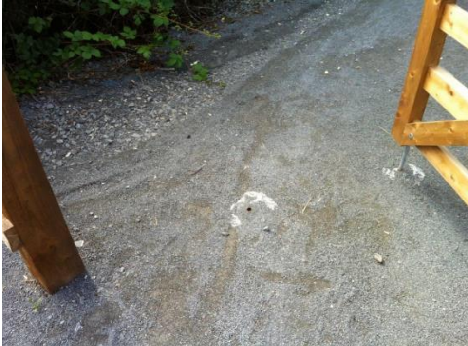
Figure 9: Greenway Gate with a second socket for the drop bolt which provides a wider opening
