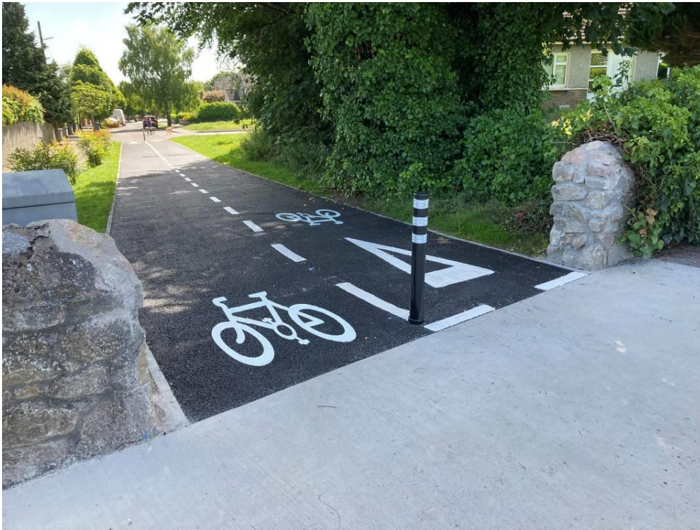
Figure 10: Wide gap with 70mm diameter bollard in the centre, with 1.5m clear space each side. (Note: Contrasting bollard colour recommended)
