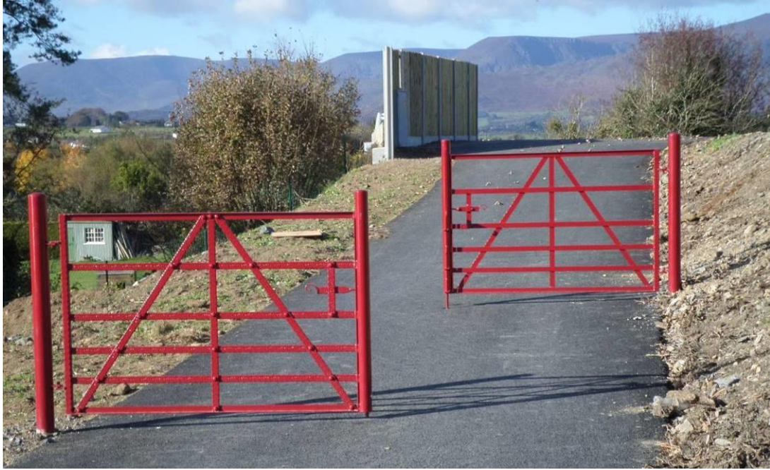
Figure 14: Example of horizontal deflection with a staggered pair of gates that also provides a distinctive visual character to a greenway.
