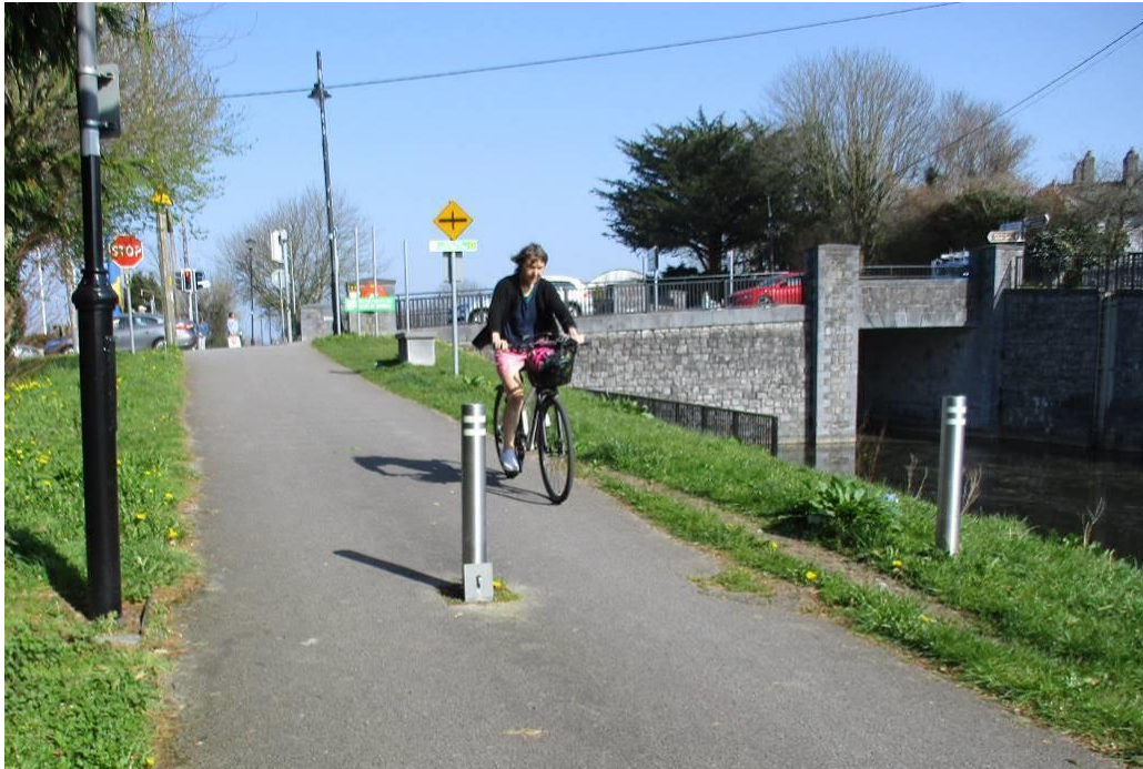
Figure 12: An example of well positioned demountable bollard using a lamp post as part of the access control arrangement. (Note: Stainless steel can be difficult to see in some conditions and is not recommended)
