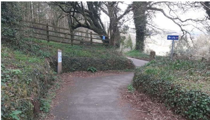
Figure 8: A change in direction on the approach to an access point onto a road. (Source: Access to Routes, Sustrans, November 2019)
