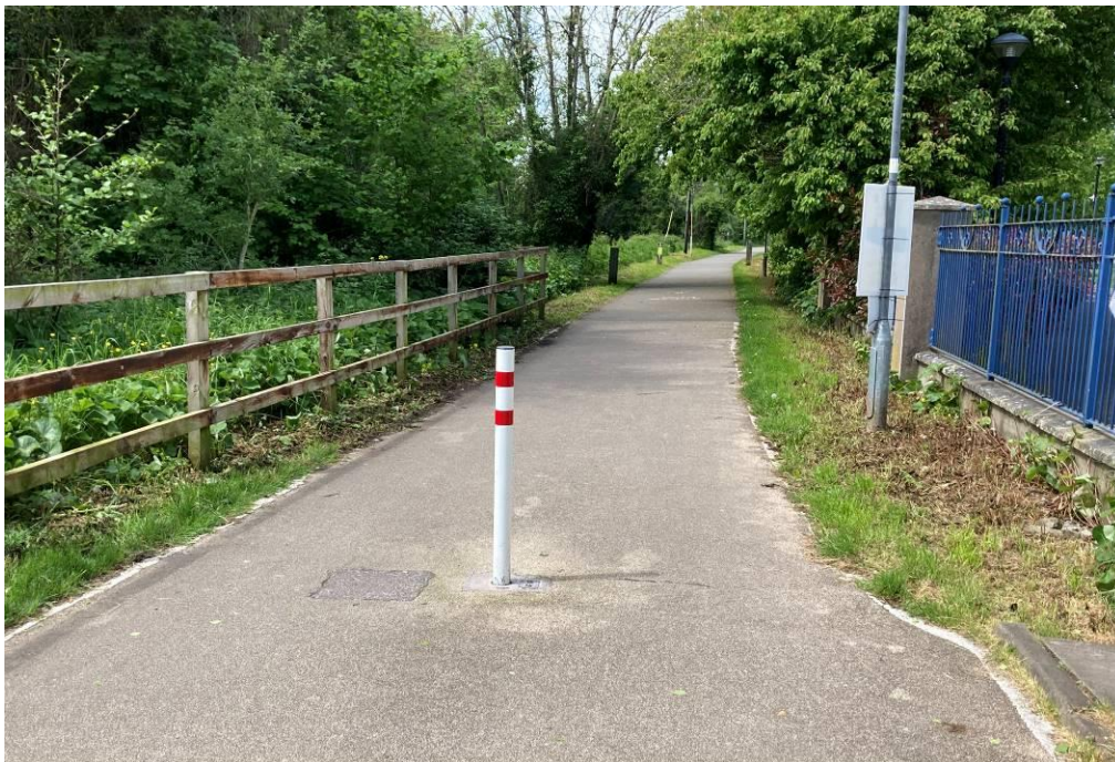
Figure 11: Optimal arrangement with brightly coloured bollard. (Note: Road markings at the base of bollard recommended)
