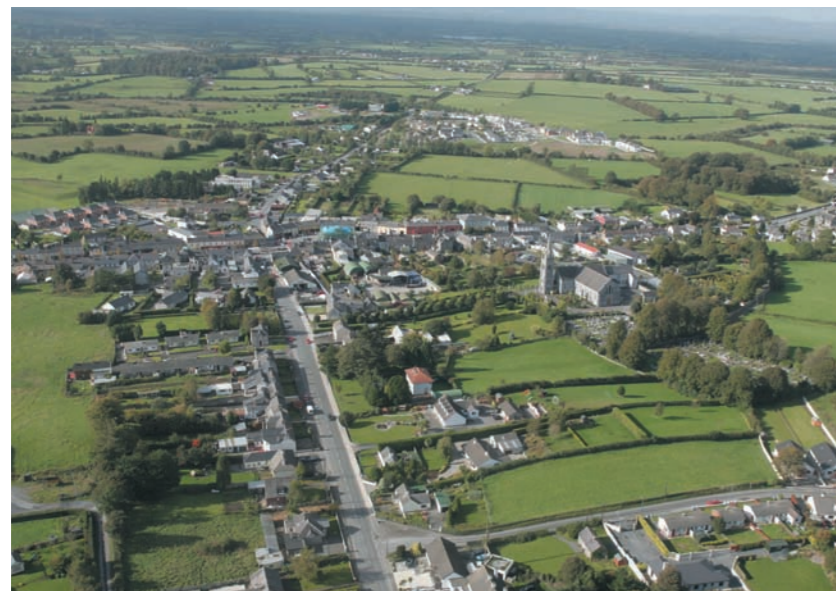
Aerial view from east
